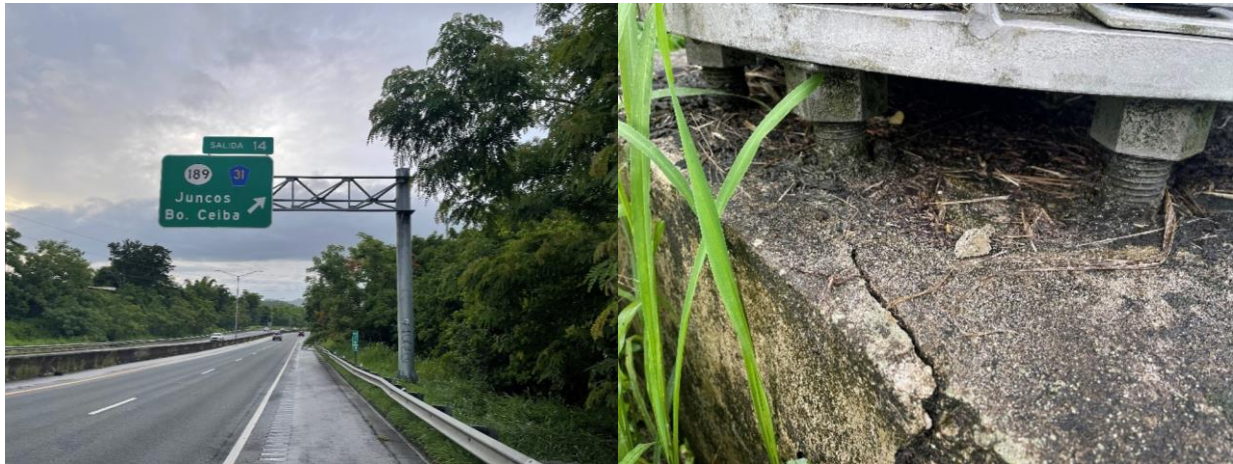
Figure 5-50: Photo of Cantilever Sign Structural Crack on the Pedestal at P-55 Location: 18.22131389°N; 65.91406944°W
