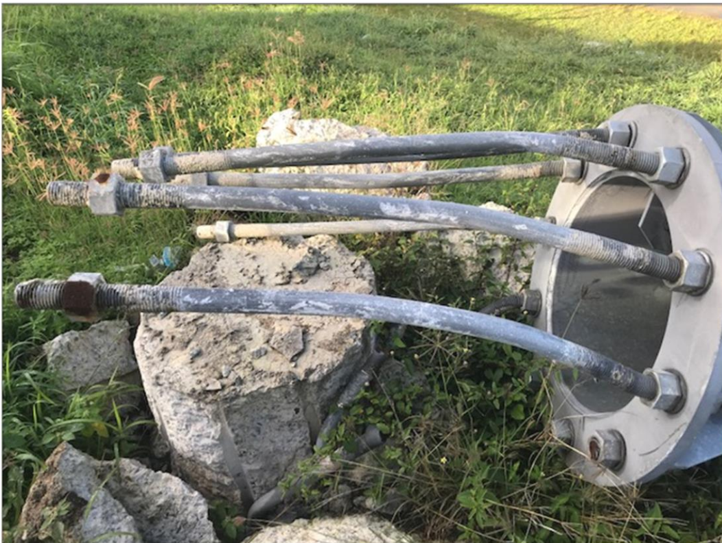
Figure 6-17: Anchor Bolts Pullout (Sign P-53)
