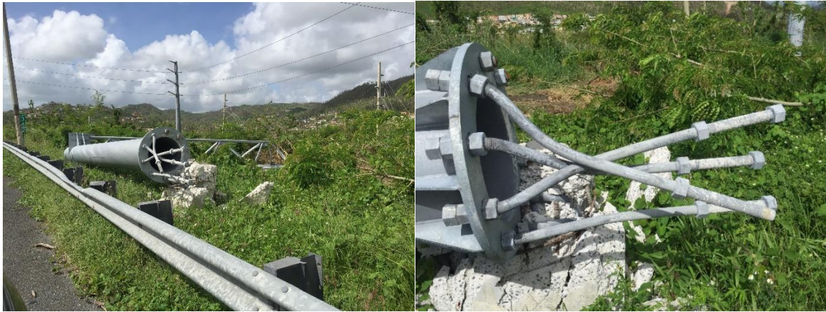
Figure 4-1: Collapsed Cantilever Sign in PR-30 Highway
