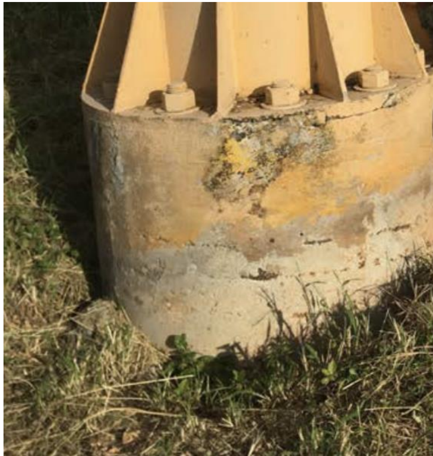
Figure 5-14: Continuous Gap Around the Circumference of the Drilled Shaft
