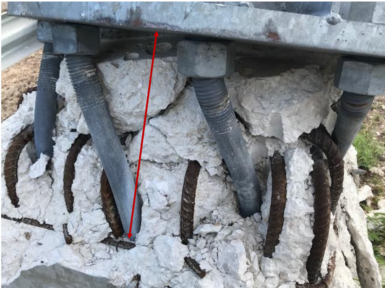
Figure 6-7: Large Deflections of Anchor Bolts due to Lack of Lateral Confinement (Sign P-46)
