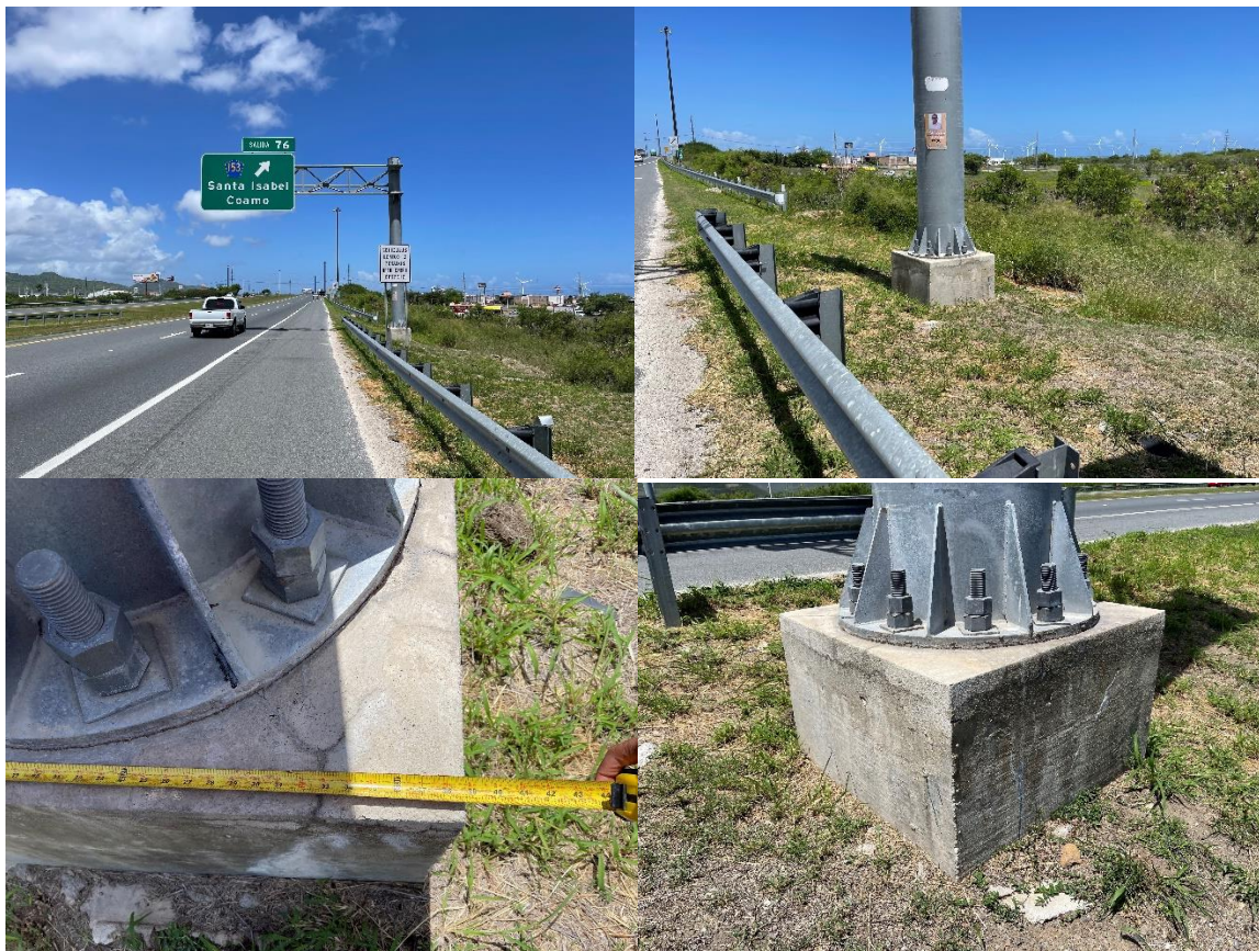
Figure 5-81: Photo of Cantilever Sign Location and Pedestal Cracks at P-8 Photo Location: 18.01293333°N; 66.389025°W
