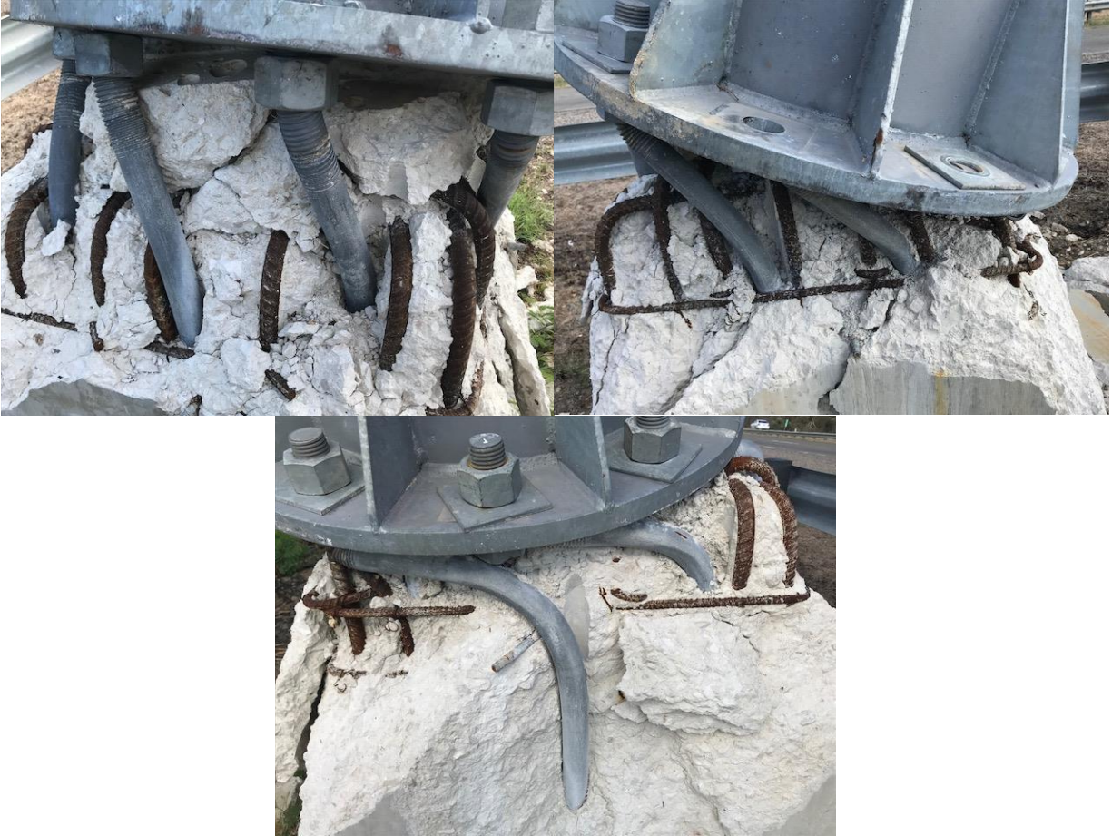
Figure 5-38: Photos of Cantilever Traffic Sign Foundation Structural Failure to the Pedestal at P-46; with Large Deflections and Bending on the Plastic Range and Shear Fracture of the Anchor Elements, and Fractures, Detachments and Crushing of the Concrete
