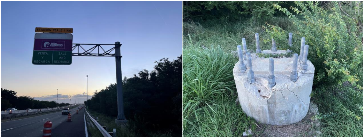
Figure 5-59: Photo of Cantilever Sign Foundation Structural Damages on the Pedestal at P-4, Damages (Fractures on the Concrete Base) Location: 17.986208°N; 66.6033°W
