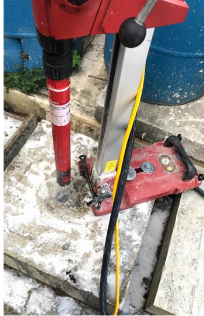
Figure 8-10 Drill Equipment Installed and Performing Extraction
