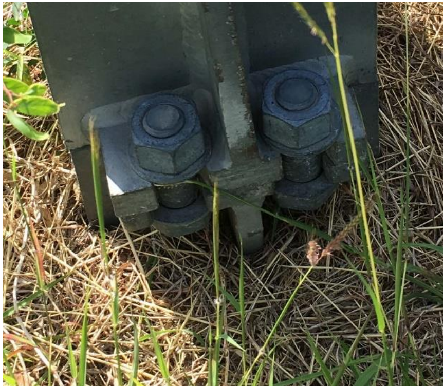
Figure 2.13: Breakaway base for unidirectional impact
