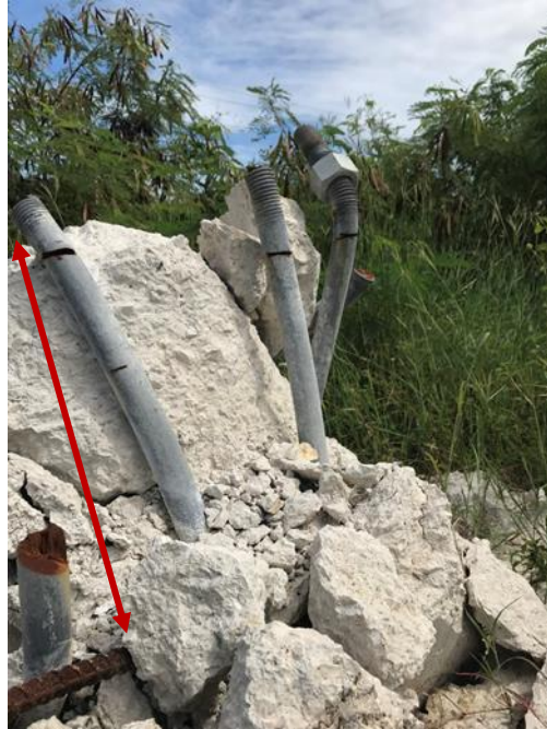
Figure 6-9: Large Deflections of Anchor Bolts due to Lack of Lateral Confinement (Sign P-12)
