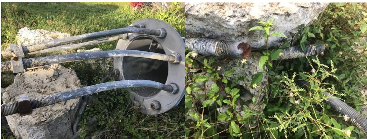
Figure 5-54: Photos of Cantilever Traffic Sign Foundation Structural Pedestal Failure at P-53; with Large Deflections on the Plastic Range, Shear Fracture, and Pullout of the Anchor Elements, and Fractures and Detachments of the Concrete
