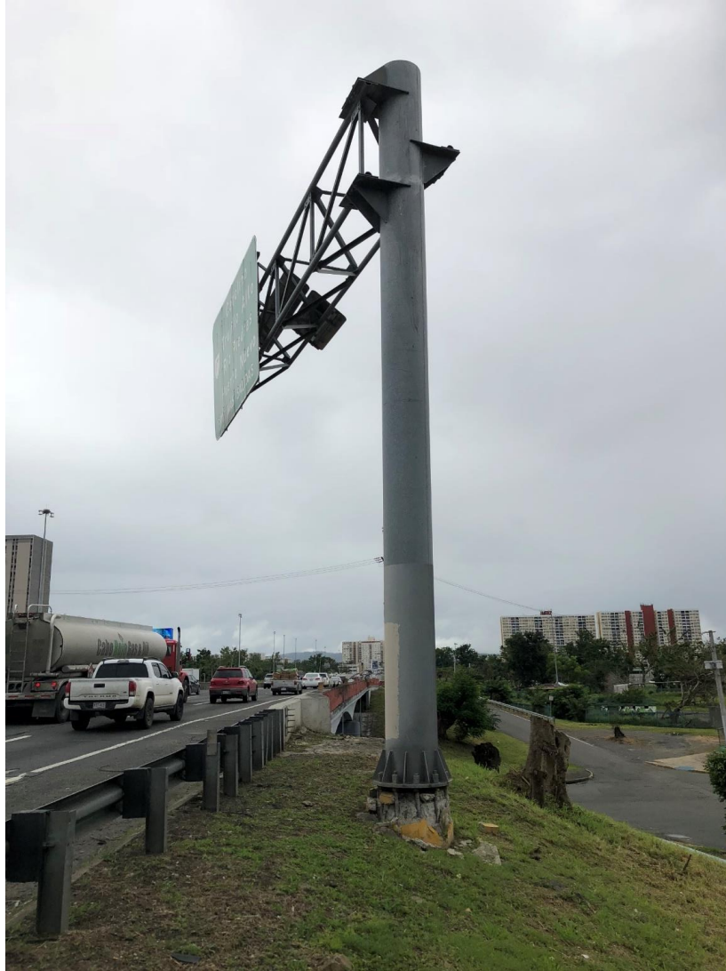
Figure 6-21: Cylindrical Precast Concrete Base that Experienced Torsional Rotation. PR 18 in San Juan
