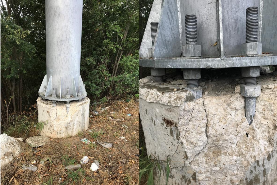
Figure 6-1: Initial Stages of Concrete Cracks and Spalls due to Lateral Deflections of Anchor Bolts (Sign P-1)
