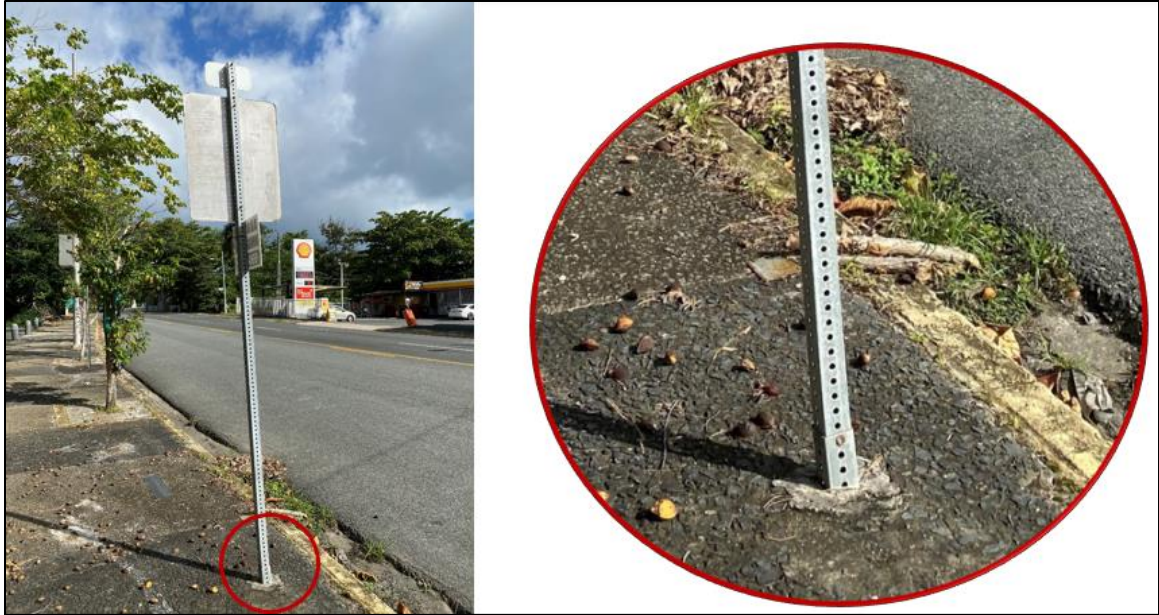
Figure 4.4: Out of plumb square tube due to construction defect
