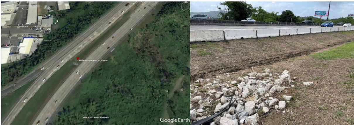
Figure 5-27: Photos of Cantilever Traffic Sign Geolocation and Rests of the Post Foundation at P-22. Location: 18.27201944N; -66.03914444W
