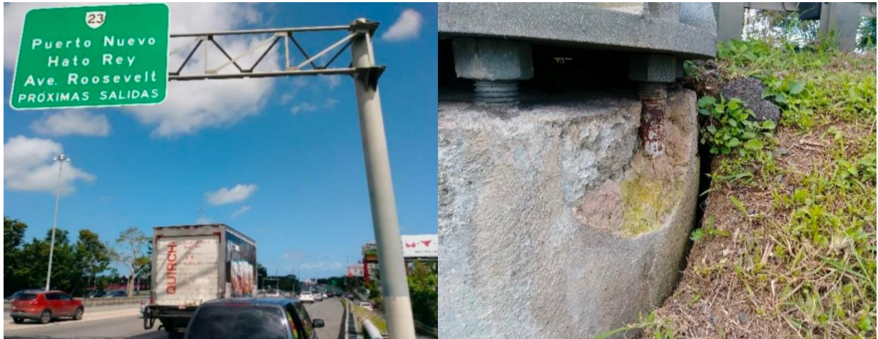
Figure 5-75: Photo of Cantilever Sign Foundation Failure (Torsional Rotation), Damages to the Concrete Pedestal, and Gap Between Soil and Shaft at P- 43 Photo Location: 18.41788611°N; 66.07006111°W
