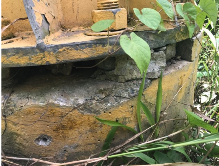
Figure 6-3: Initial Stages of Concrete Cracks and Spalls due to Lateral Deflections of Anchor Bolts (Sign P-76)
