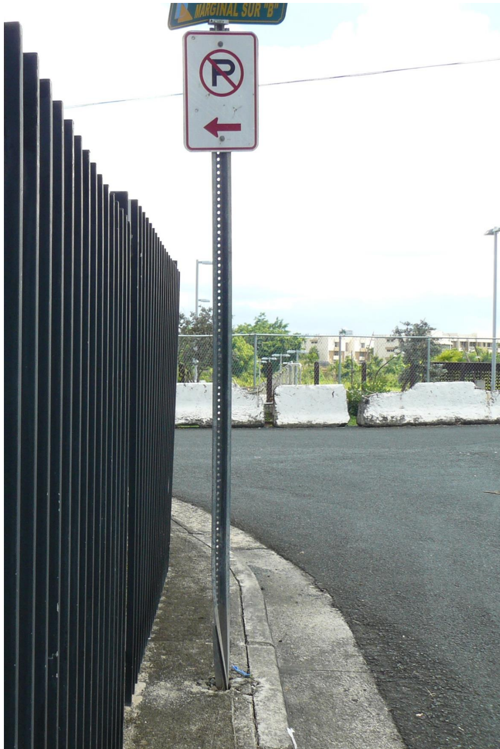
Figure 4.11: Sign facing wrong direction due to permanent twisting deformation
