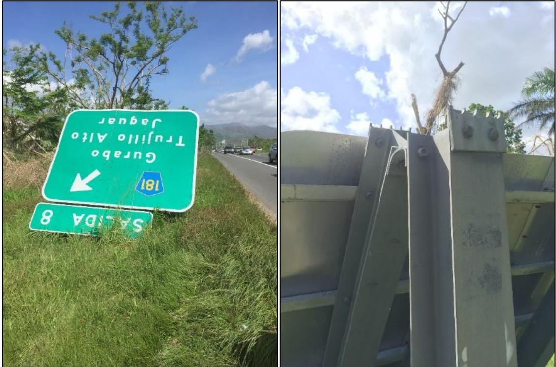
Figure 4.8: Fuse plate rupture of Case 2
