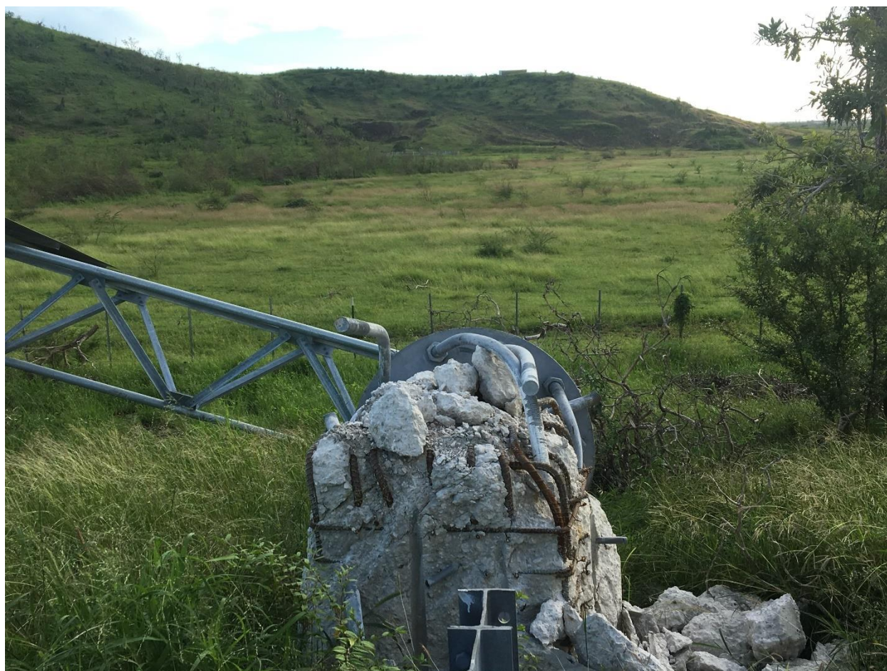
Figure 6-13: Some of the Anchor Bolts Outside the Transverse Confinement Steel / Concrete Core (Sign P-100)
