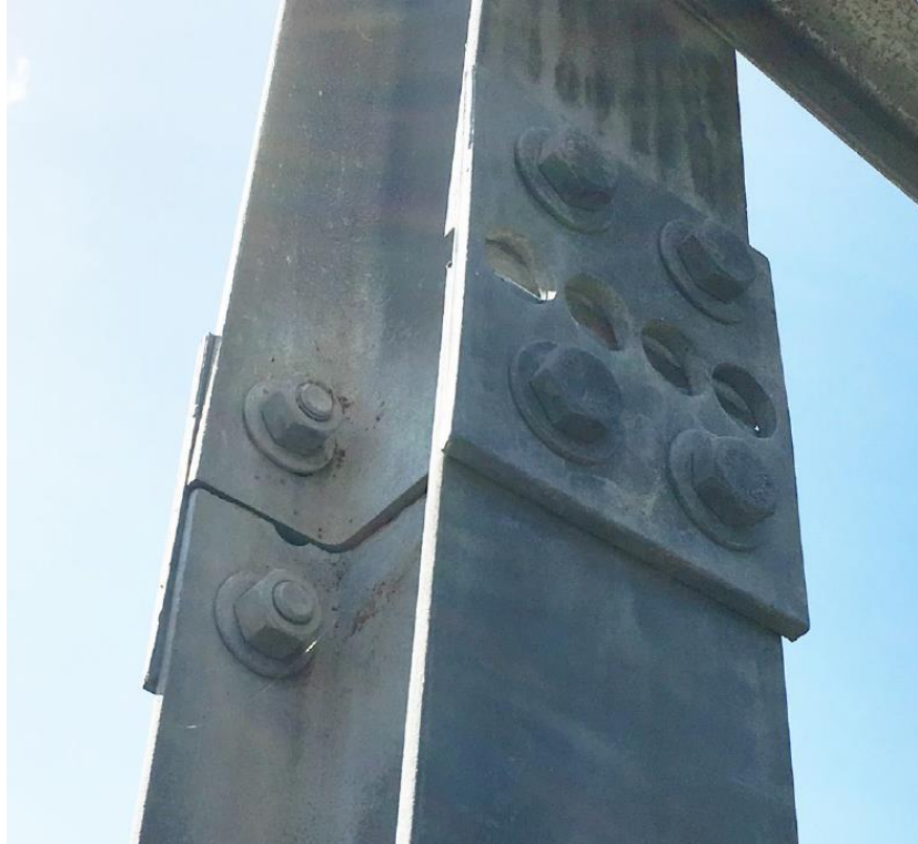
Figure 2.9: Fuse plate
