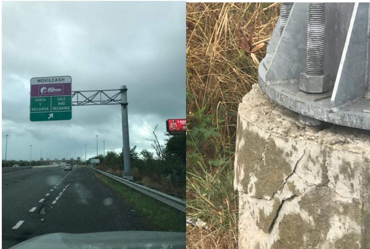
Figure 5-58: Photo of Cantilever Sign Foundation Structural Damages on the Pedestal at P-3, Damages (Fractures on the Concrete Base) Location: 17°59'19.75"N; 66°37'0.41"W
