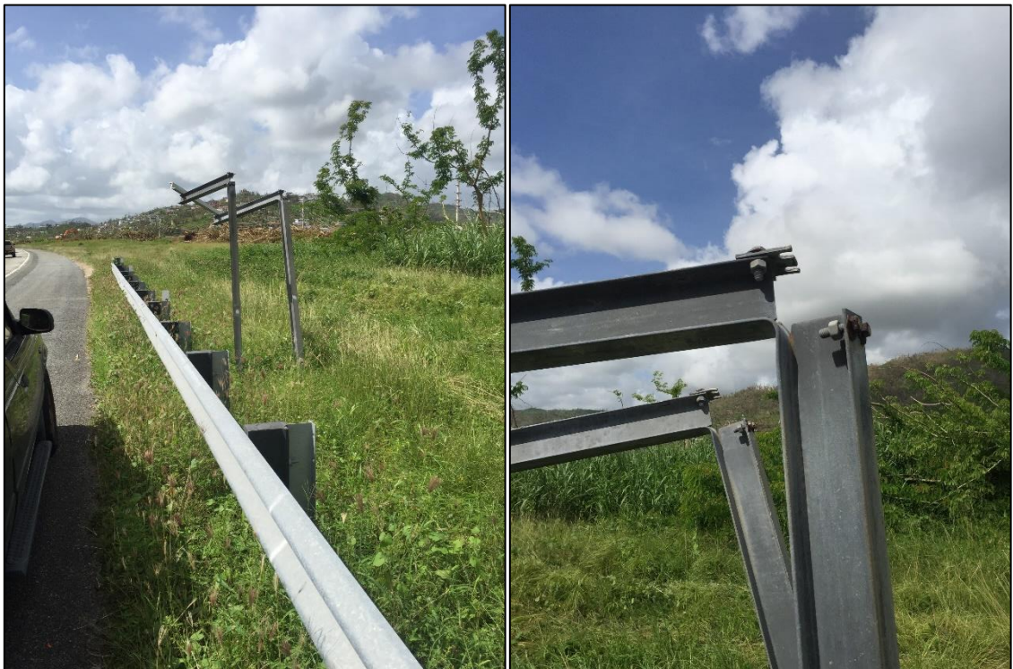
Figure 4.10: Undetermined mode of failure of Sign 10
