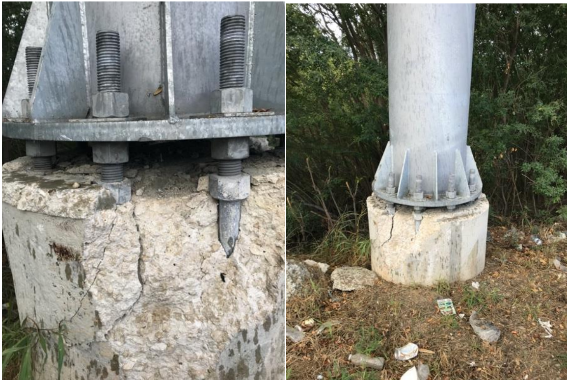
Figure 5-57: Photo of Cantilever Sign P-1. Damages, Fractures on Concrete Pedestal. Location: 17°59'25.25"N; 66°37'16.63"W
