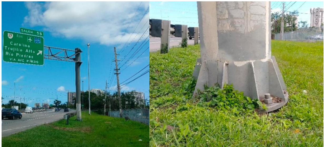
Figure 5-69: Photo of Cantilever Sign Soil Foundation Failure (Torsional Rotation) at P- 35 Photo Location: 18°24'16.37"N; 66° 4'11.96"W
