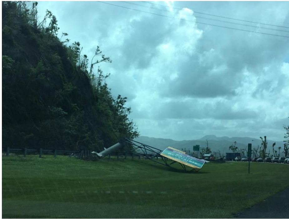
Figure 6-23: Foundation that Experienced Torsional Rotation and Overturning. PR 52 in Caguas.
