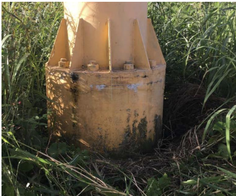
Figure 5-9: Photo of Drilled Shaft Foundation of Traffic Sign P-77
