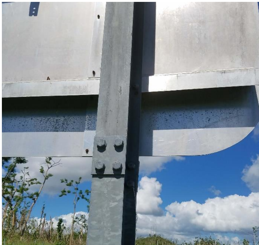
Figure 2.10: Hinge plate
