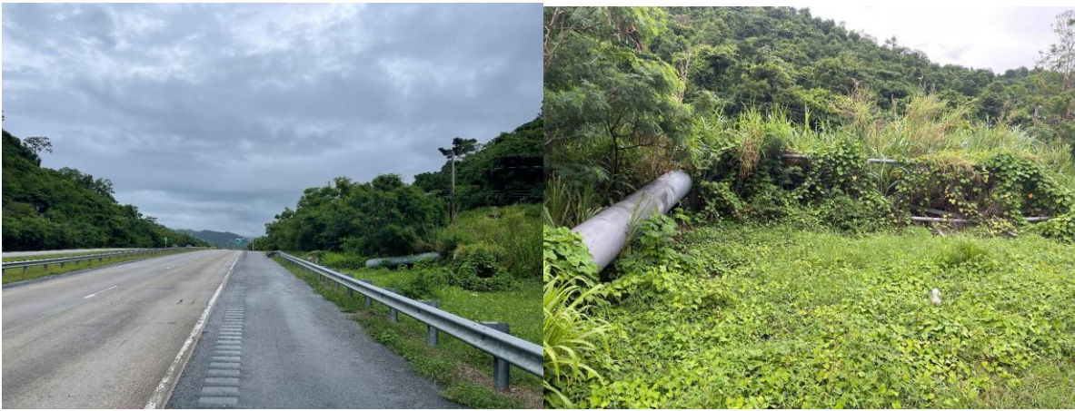
Figure 5-42: Photo of Cantilever Sign Foundation Structural Failures on the Pedestal and Sign Position (Total Collapse) at P-61. Location: 18.159975°N; 65.79745833° W
