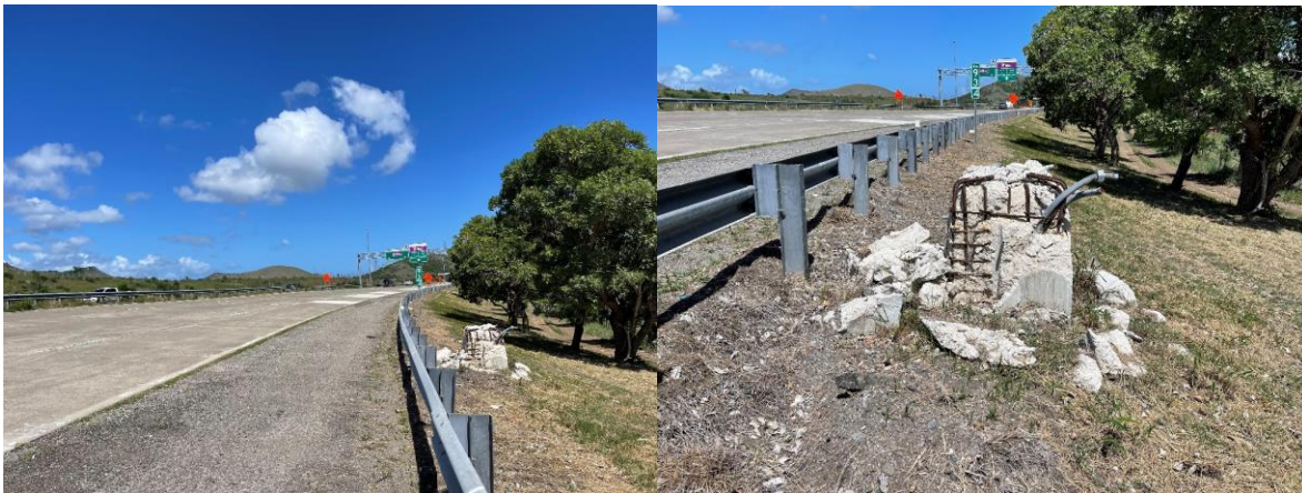
Figure 5-64: Photo of Cantilever Sign Structural Failures on the Pedestal at P-12 Location: 18° 0'11.23"N; 66°14'29.63"W
