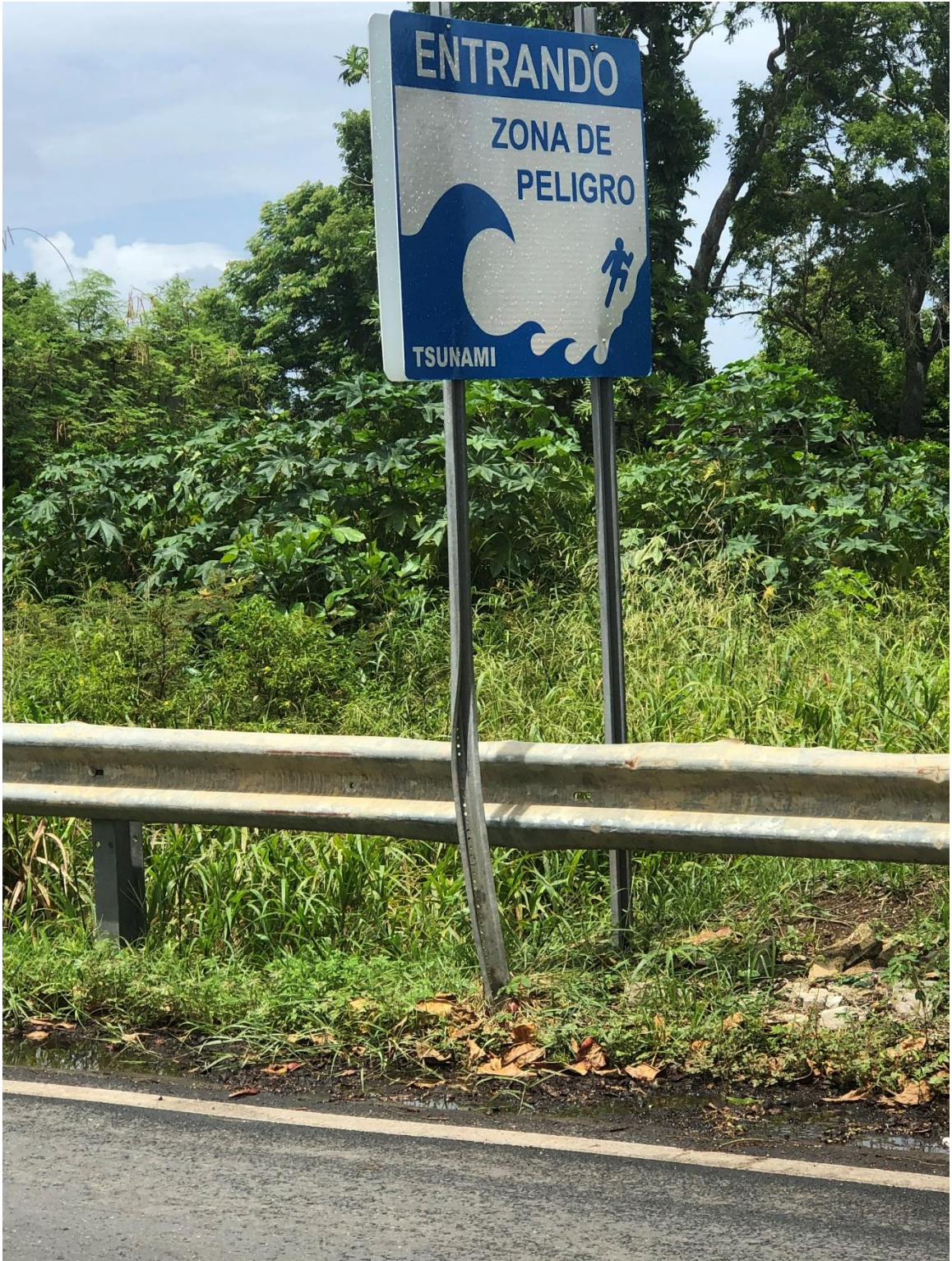
Figure 4.15: Sign with multiple U-channel posts where one post experienced permanent twisting deformation
