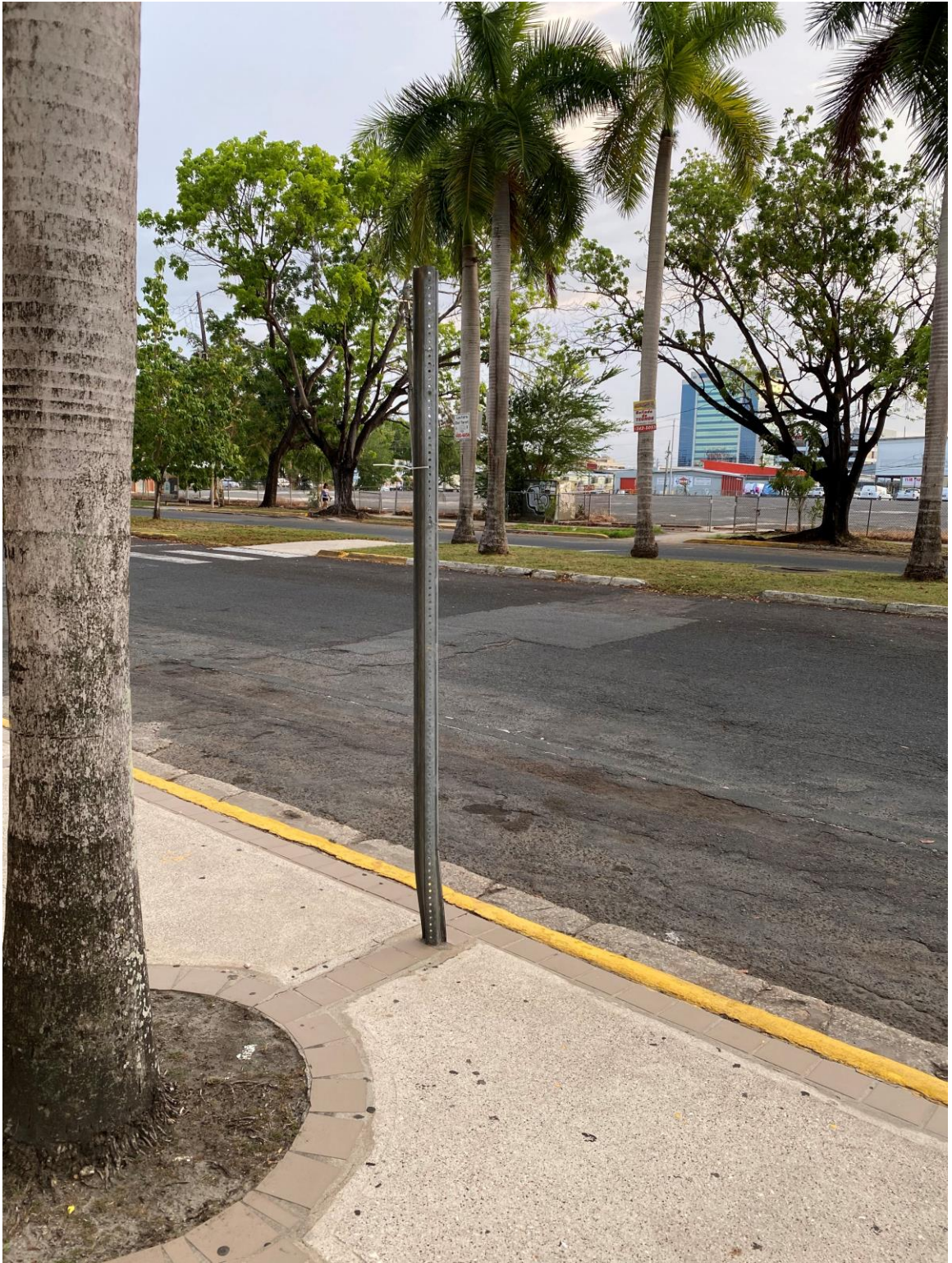
Figure 4.12: Permanent twisting deformation post that lost sign panel
