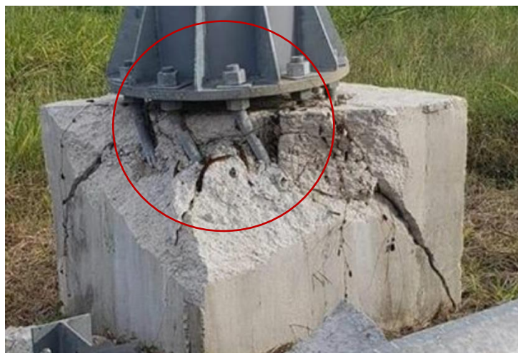
Figure 6-6: More Advance Stage of Concrete Cracks and Spalls due to Lateral Deflections of Anchor Bolts with Large Unconfined Length. Bolts Exhibit Double Bending Shape (Sign P-15)
