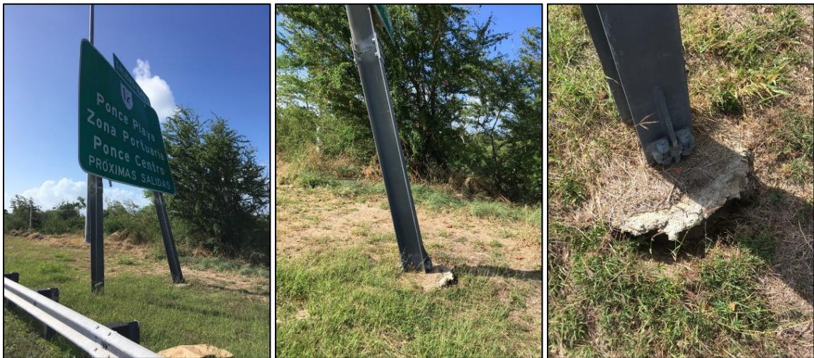
Figure 4.2: Foundation failure of Sign 6
