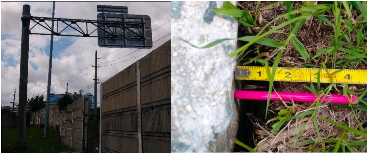
Figure 5-68: Photo of Cantilever Sign Foundation Soil Failure (Torsional Rotation) at P- 33 Photo Location: 18°23'52.03"N; 67° 66° 4'14.19"W
