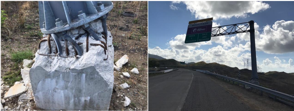
Figure 5-37: Photo of Cantilever Sign Foundation Structural Failures on the Pedestal and Sign Position (Partial Collapse) at P-46. Location: 17°59'8.91"N; 66° 8'45.56"W
