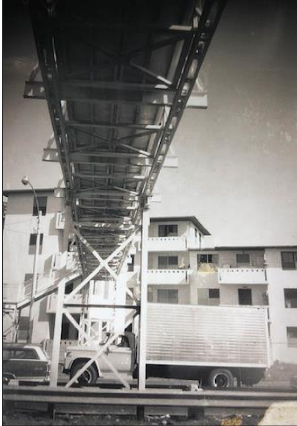
Figure 5.52: Underside and north end of PB 1307 taken between 1968 and 1990 (Source: PRHTA)
