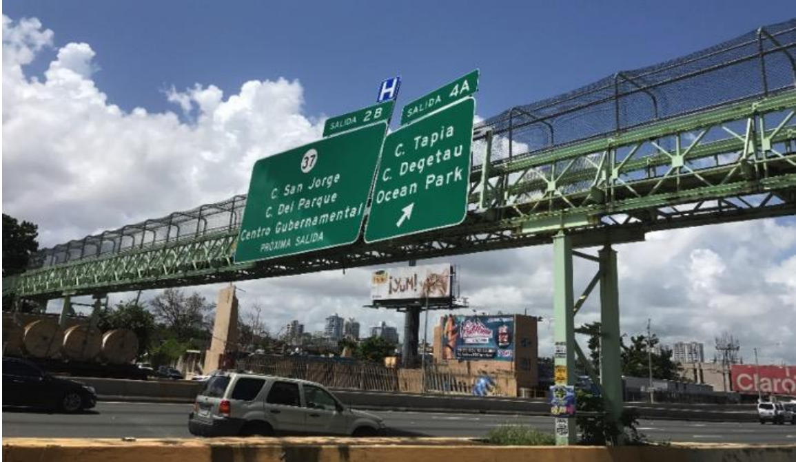
Figure 4.3: Image of the Bridge from September 2018 (Provided by PRHTA)
