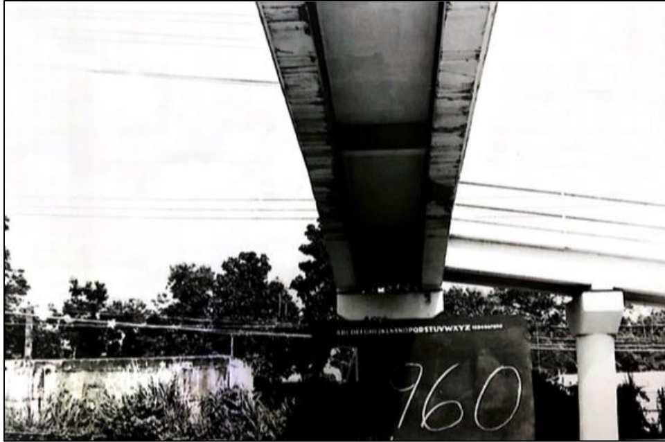
Figure 5.7: Underside of PB 0960 on July 21, 1972 (Source: PRHTA)
