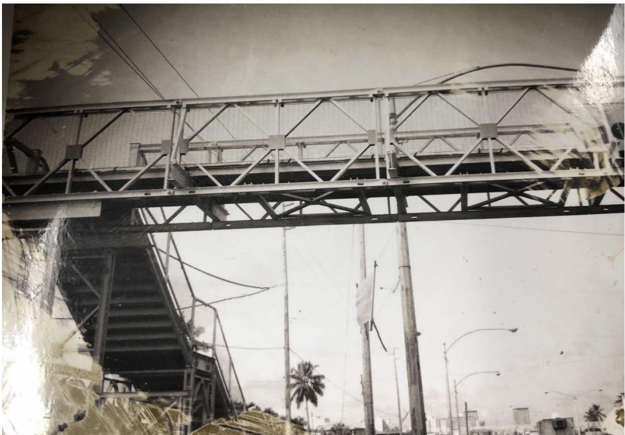
Figure 5.51: Photo of south end of PB 1307 taken between 1968 and 1990 (Source: PRHTA)
