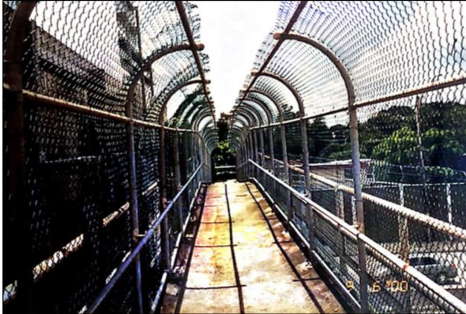
Figure 5.9: Walkway of PB 0960 on September 6, 2000 (Source: PRHTA)
