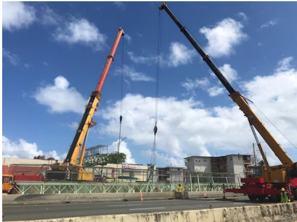
Figure 7.2: Bridge Being Removed
