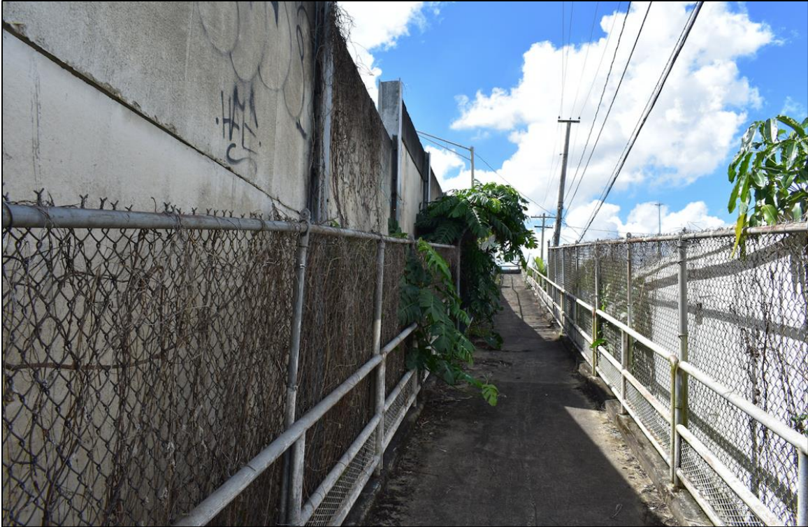
Figure 5.14: Vegetation in chain-link fencing
