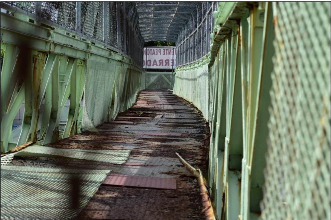
Figure 5.41: Curvature in deck
