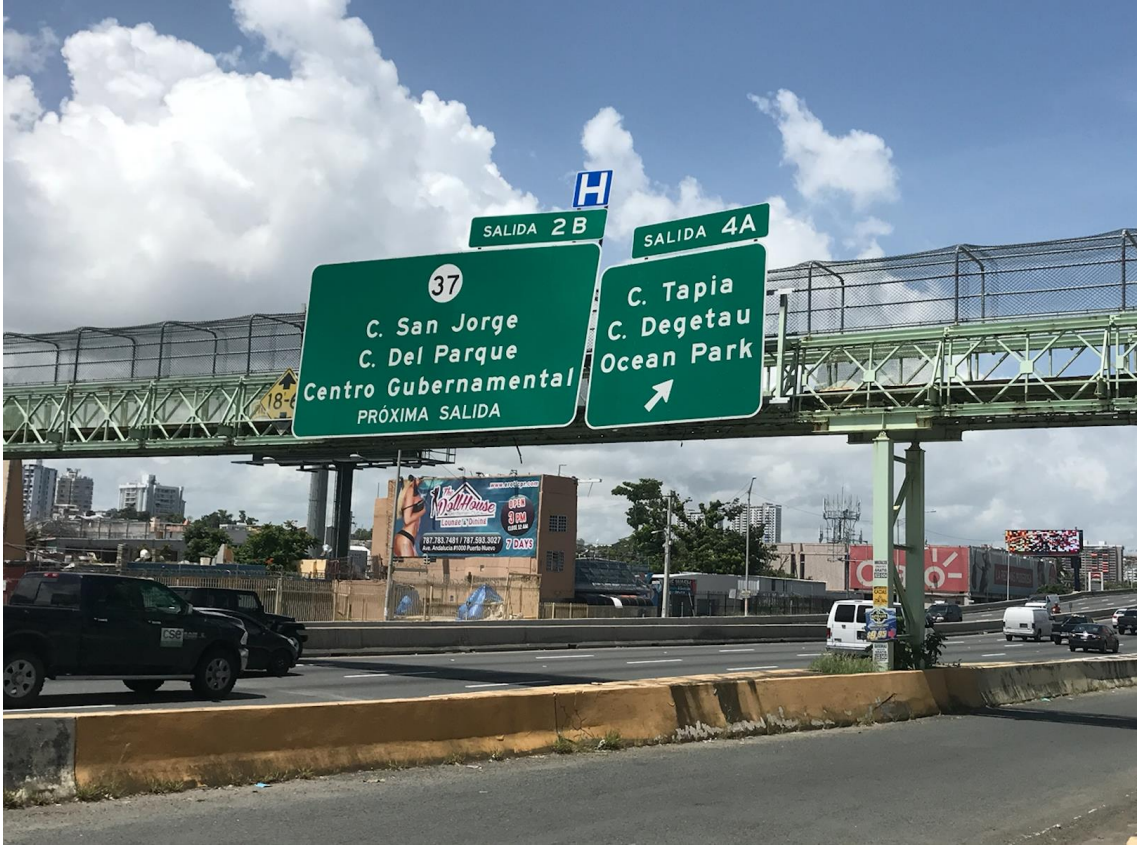
Figure 8.8: Signage Installed at the Pedestrian Bridge
