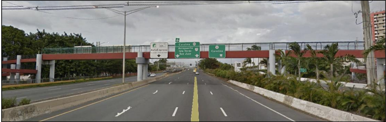
Figure 5.66: Pedestrian Bridge 2336 (Source: Google Earth Pro)
