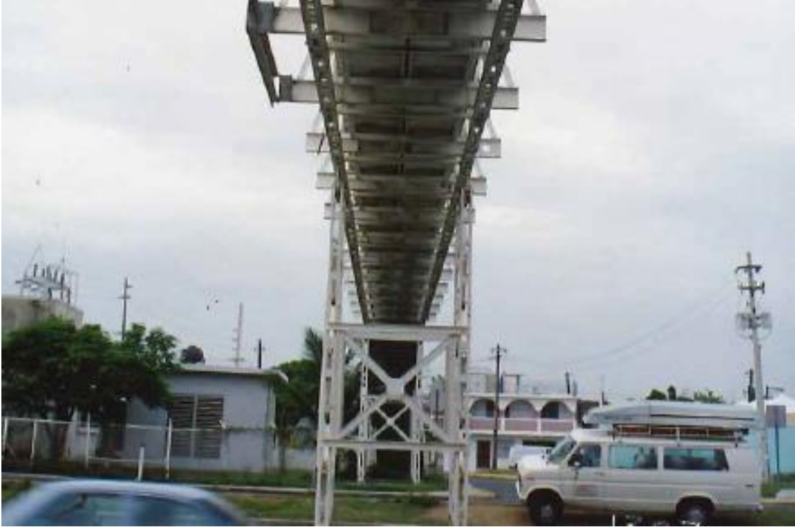
Figure 5.59: Underside of PB 1307 before Hurricane Maria (September 24, 1993) (Source: PRHTA)
