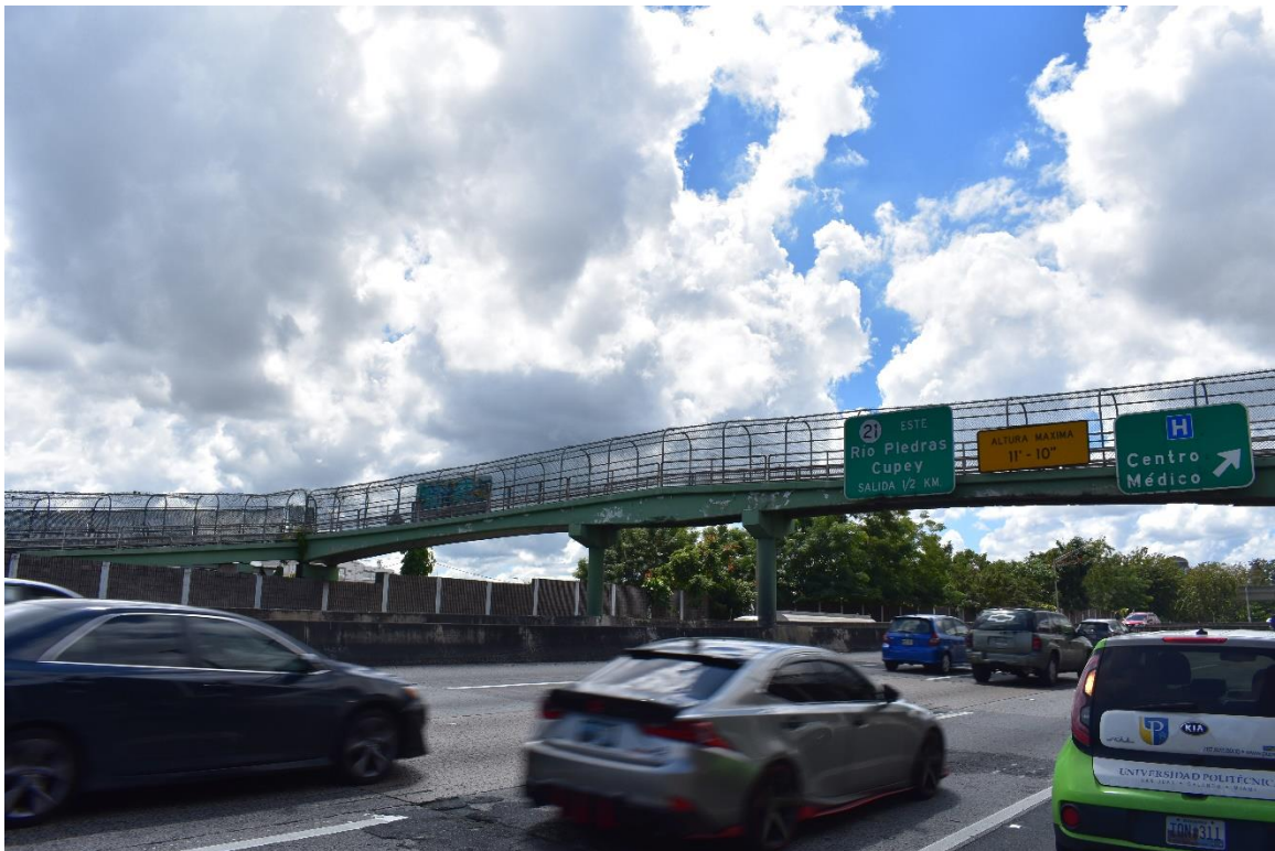
Figure 5.2: North view of PB 0960
