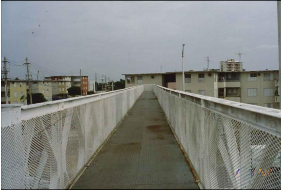
Figure 5.54: Photo of deck of PB 1307 taken on September 24, 1993 (Source: PRHTA)
