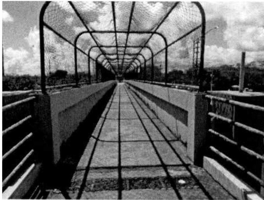
Figure 5.71 Walkway of PB 2336 on April 16, 2014 (Source: PRHTA)
