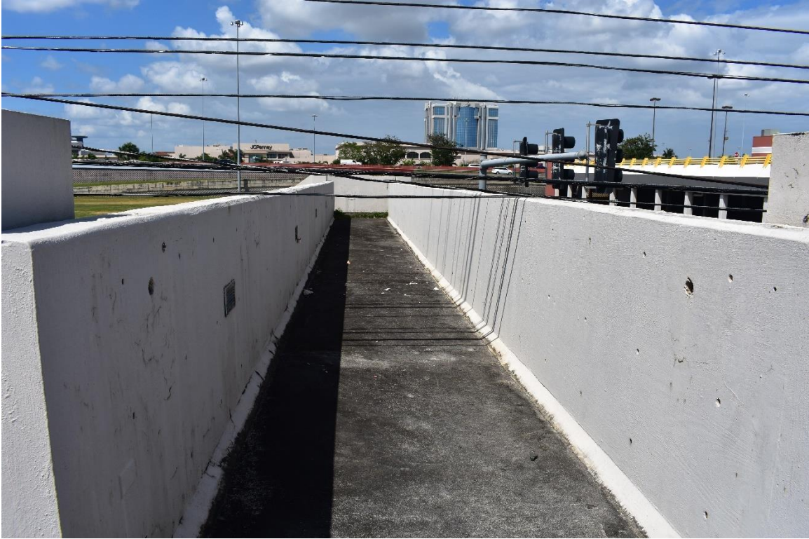
Figure 6.29: Electrical cables blacking pathway and mold and silt on PB 1926
