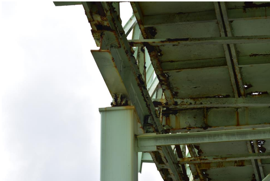
Figure 8.15: Twisted Pin-Plate and Supporting Beam
