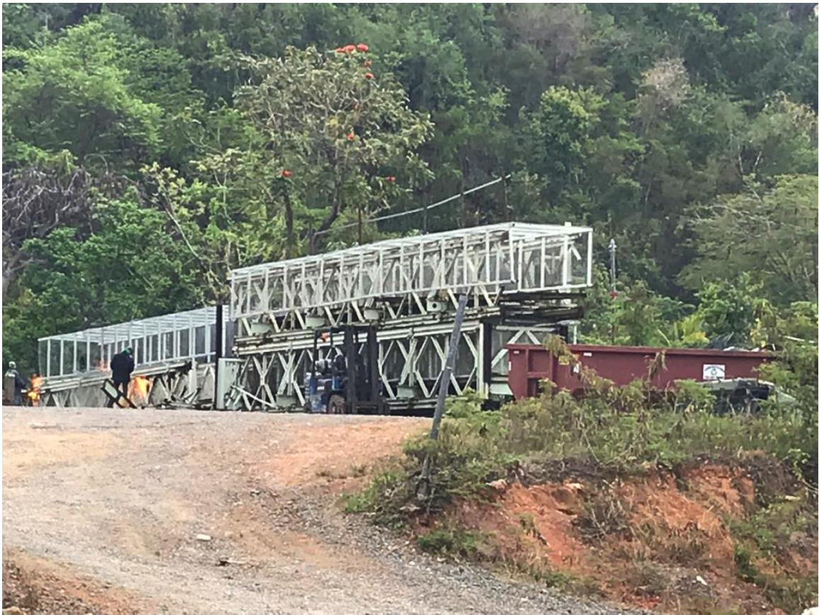
Figure 7.4: Demolished Bridge at Junkyard (April 26, 2019)
