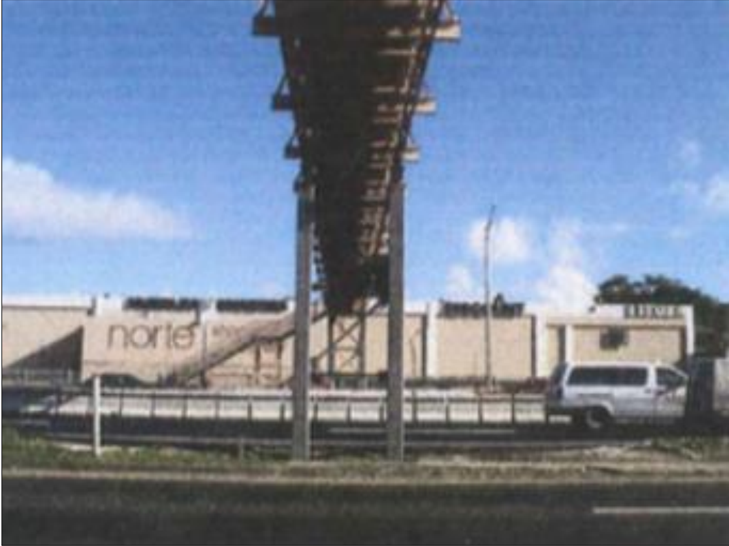
Figure 5.36: Underside of PB 1137 before Hurricane Maria (March 5, 1999) (Source: PRHTA)
