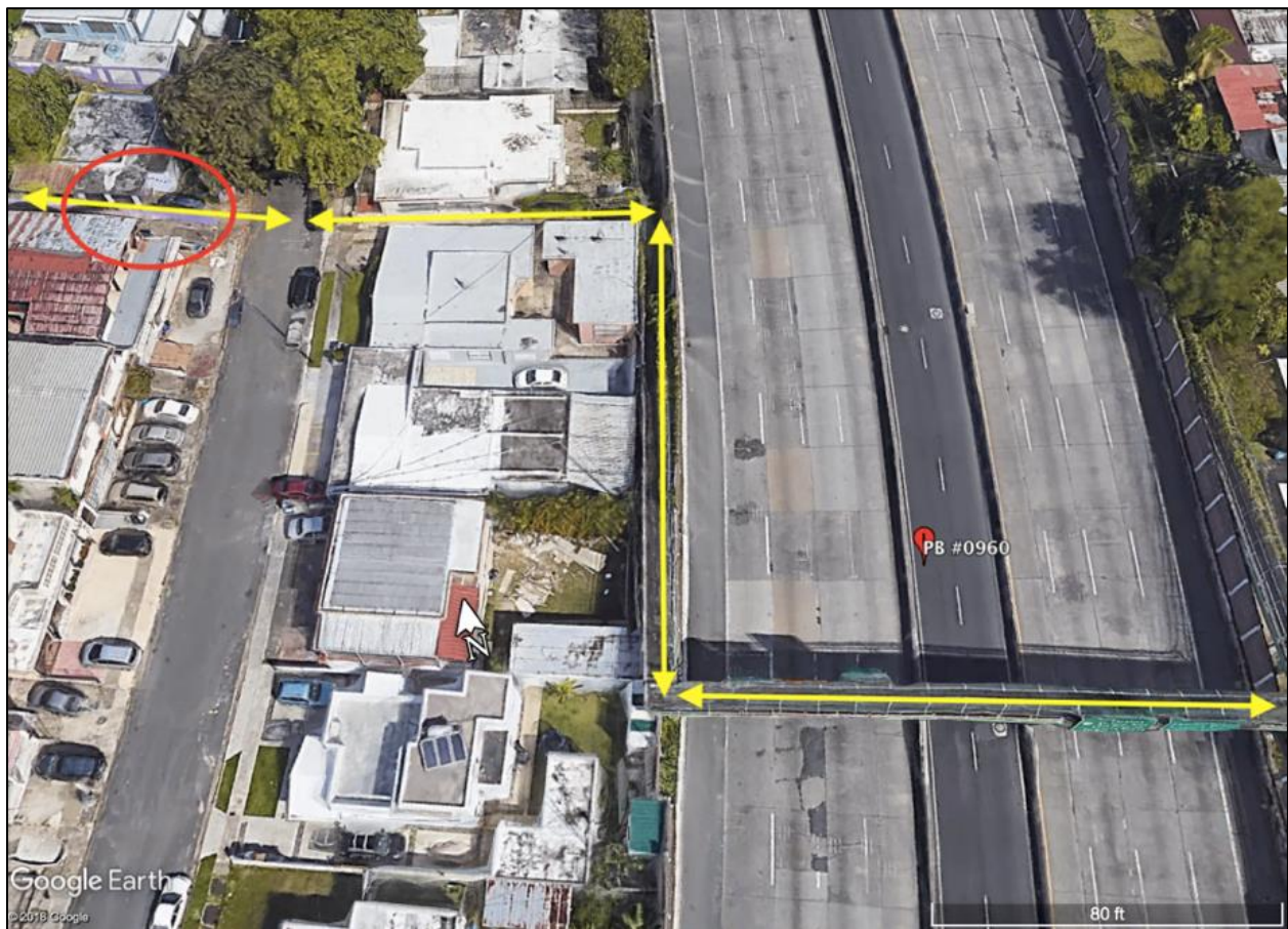
Figure 5.11: Pedestrian path with the red circle indicating location of tripping hazards (Source: Google Earth Pro)
