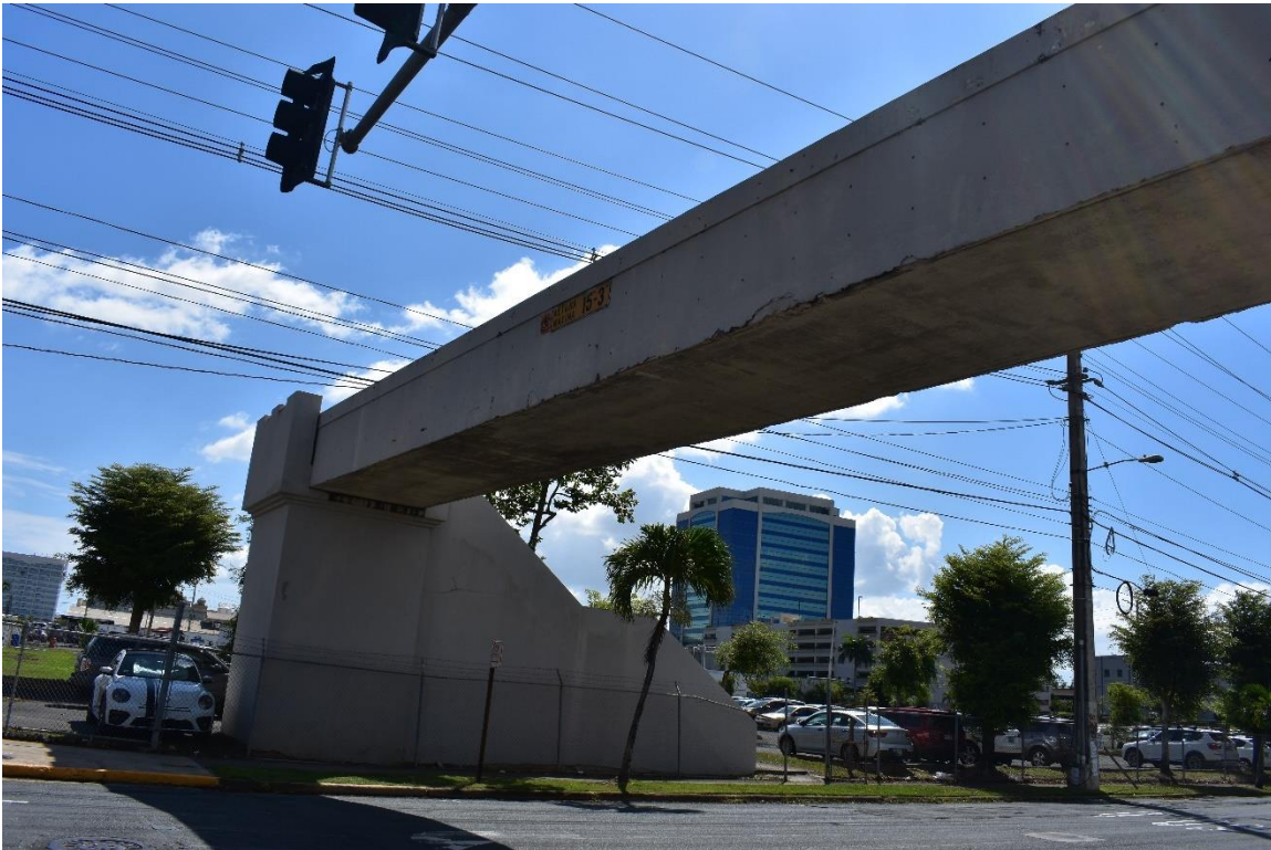
Figure 6.28: Electrical cables passing closely over PB 1926
