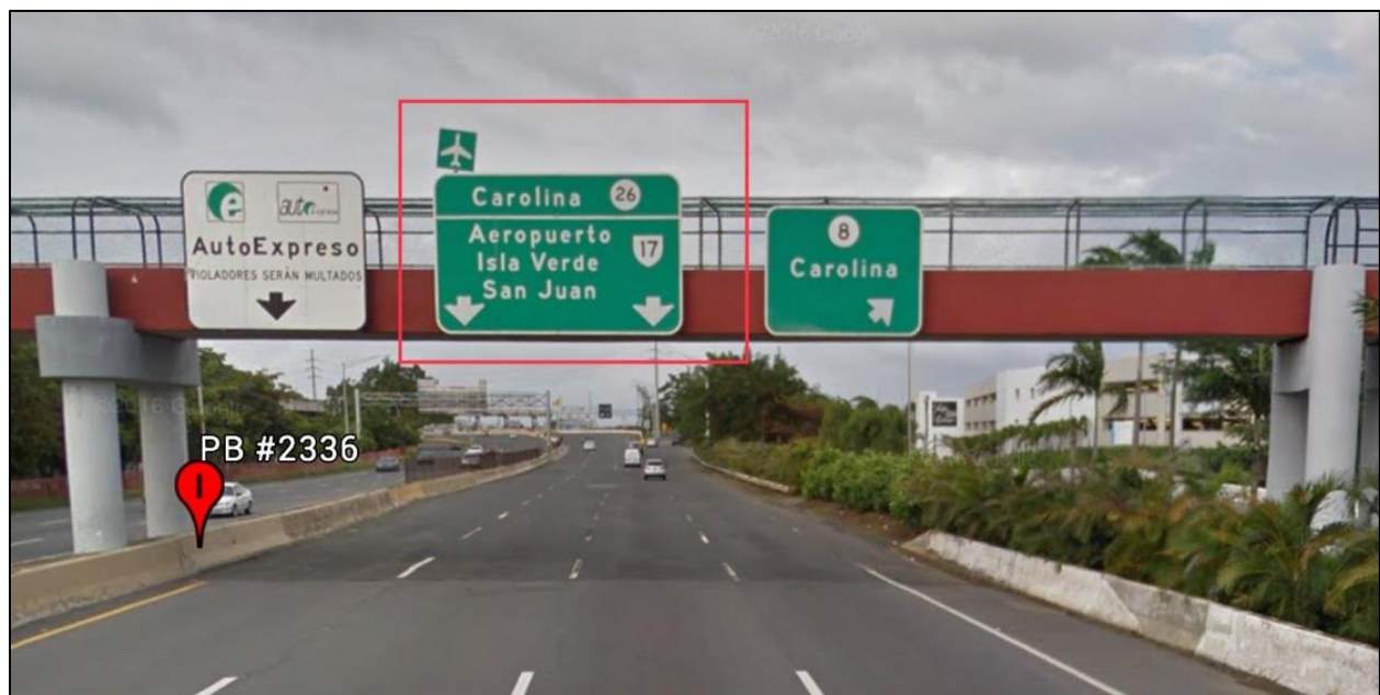
Figure 5.73: Transit Signs in south side of PB 2336 (Source: Google Earth Pro)
