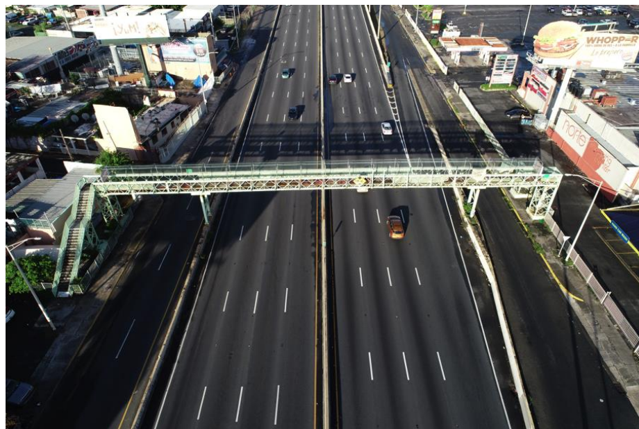
Figure 5.6: Aerial Photograph of the Pedestrian Bridge
