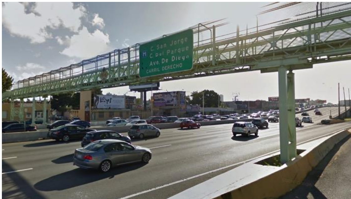
Figure 4.2: Image of the Bridge from March 2016 (Source: Google Maps)
