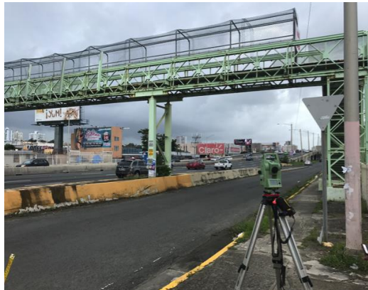
Figure 5.4: Total Station Positioned to Measure Bridge
