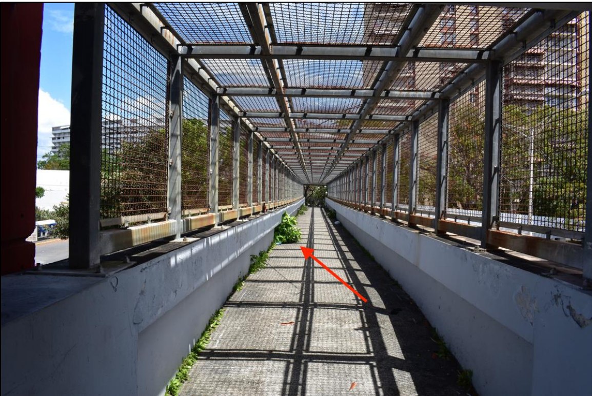
Figure 6.36: Vegetation covered drains on PB 2566
