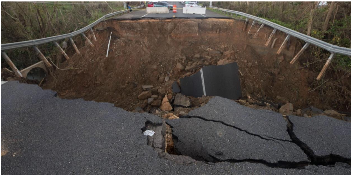
Figure 2-335: Collapsed Bridge 1733 image from news report (source: El Nuevo Día)
