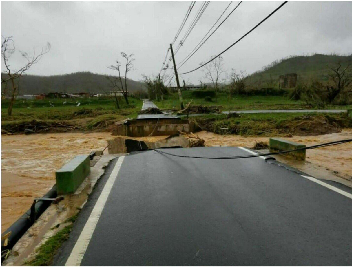
Figure 2-39: Social media image of collapsed Bridge 653 (source: L. Anqueira)
