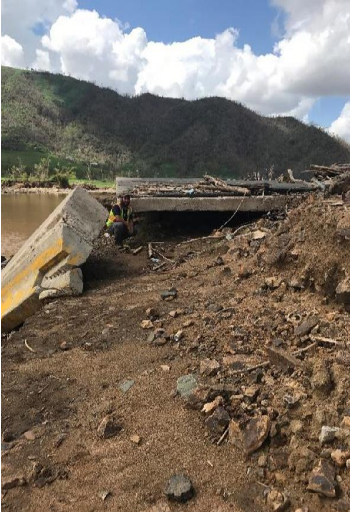
Figure 2-222: Inspection of collapsed Bridge 1462 (source: PRHTA)
