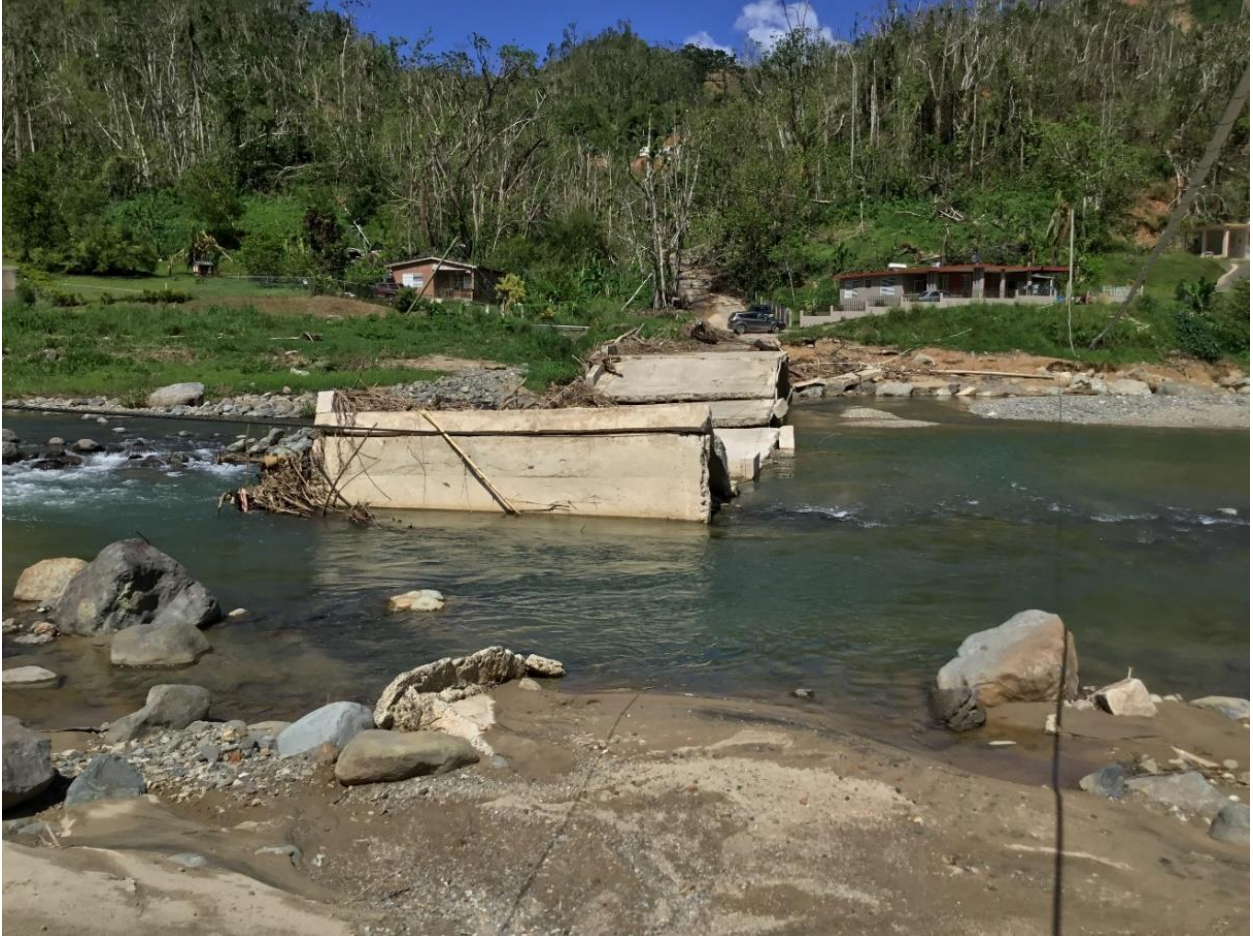
Figure 2-160: Image of collapsed Bridge 1355 (source: FHWA)
