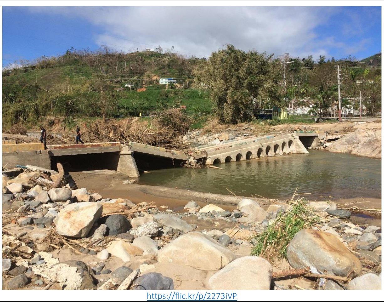
Figure 2-20: Social media image of collapsed Bridge 505 (source: Julia Maldonado)
