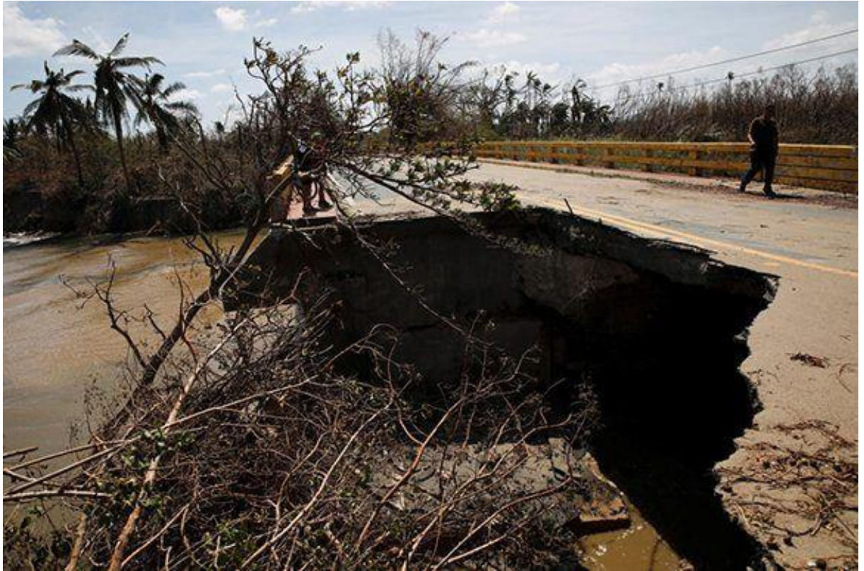
Figure 3-25: News report image of partial collapse of approach of Bridge 635 (source: Cuba Debate)
