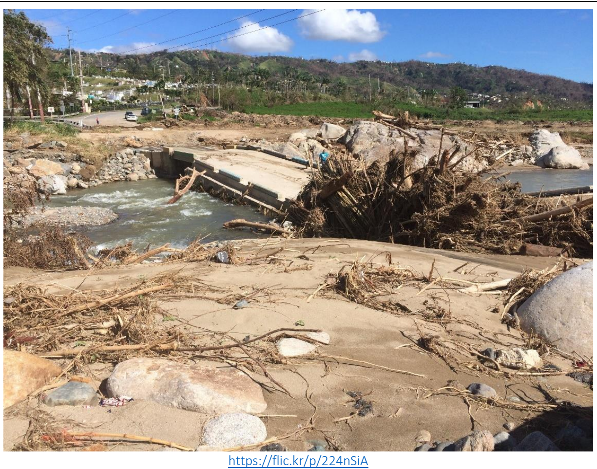
Figure 2-19: Social media image of collapsed Bridge 505 (source: Julia Maldonado)
