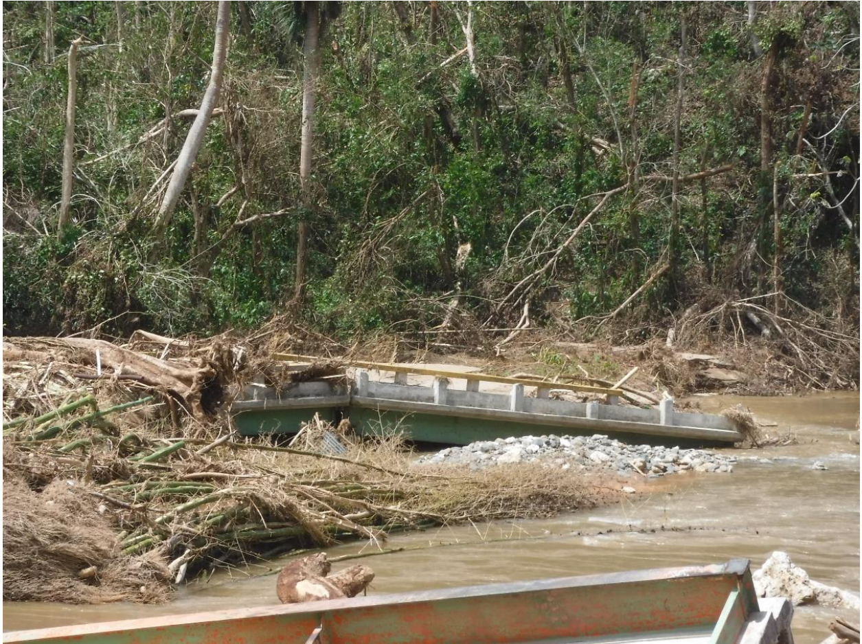
Figure 2-142: Image of deck of Bridge 505 washed down the river (source: PRHTA)
