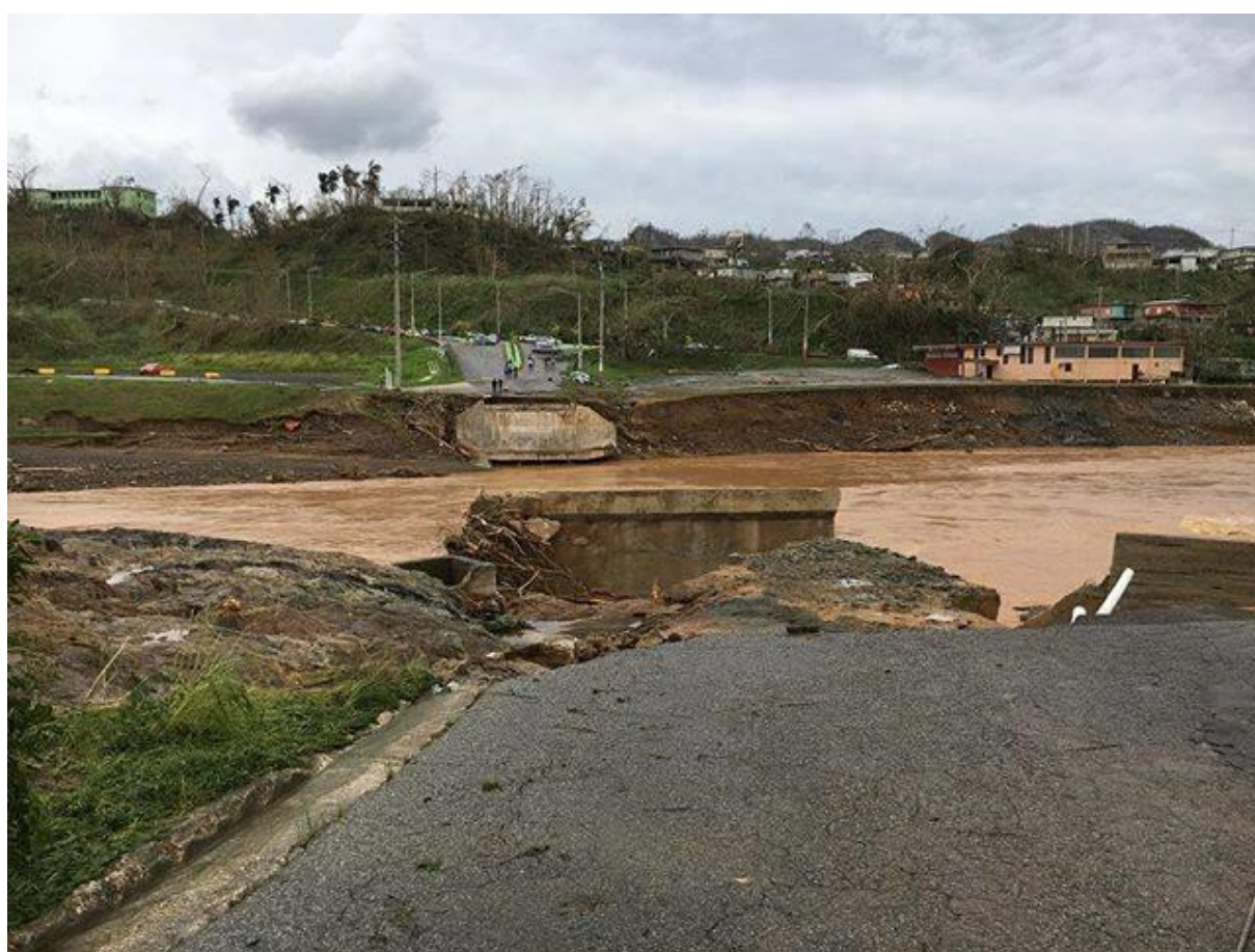
Figure 2-115: Social media image of collapsed Bridge 1130 (source: Jay Fonseca)
