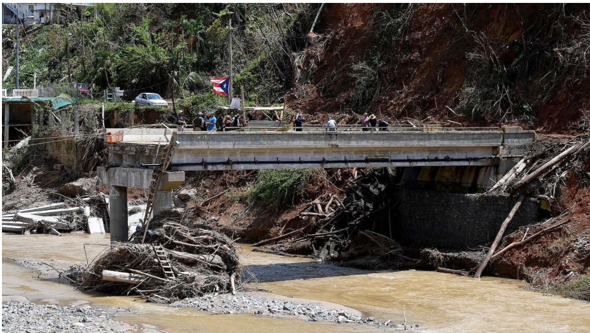
Figure 2-267: News report image of collapsed Bridge 1499 (source: Noticel)
