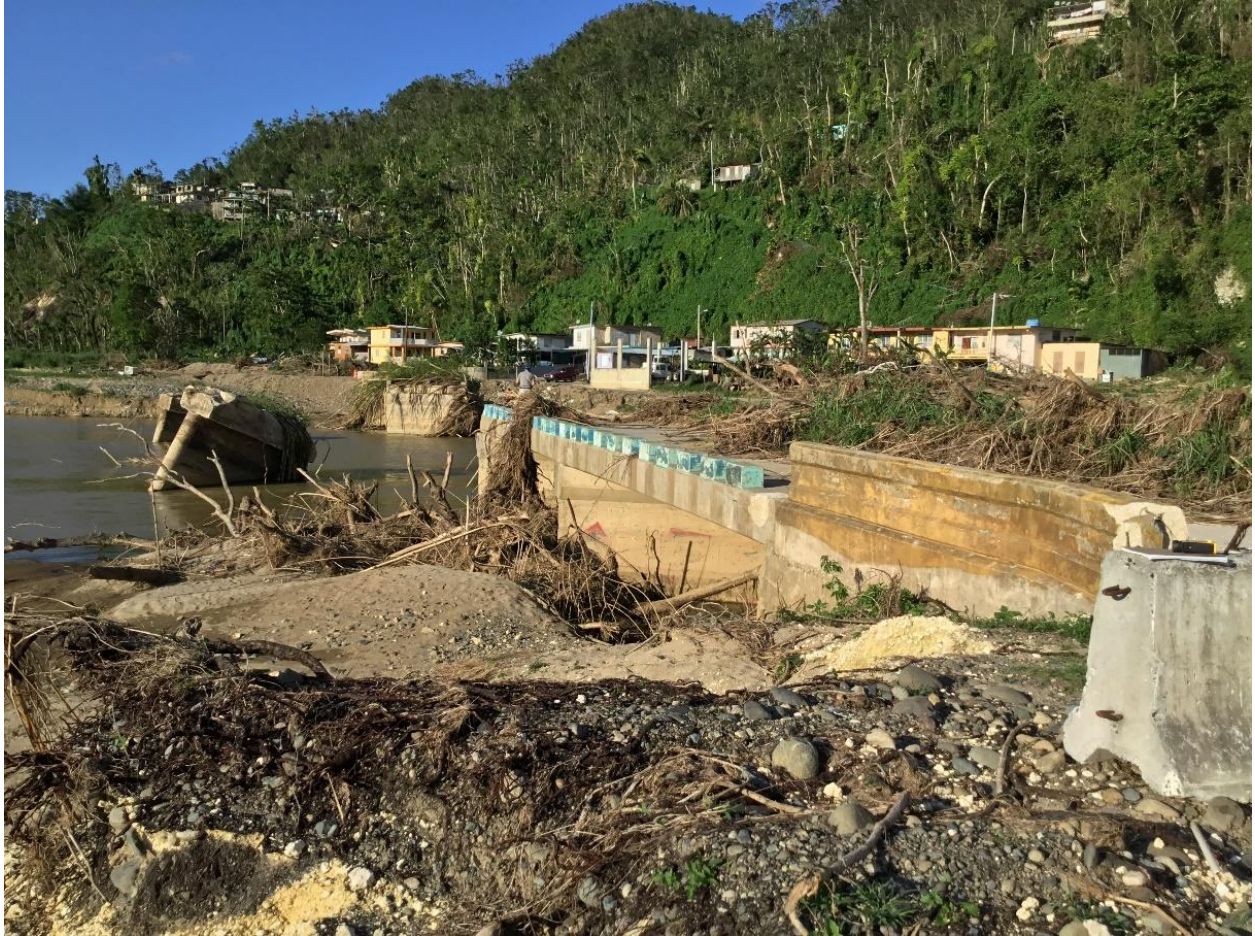
Figure 2-355: Collapsed Bridge 1917 (source: PRHTA)
