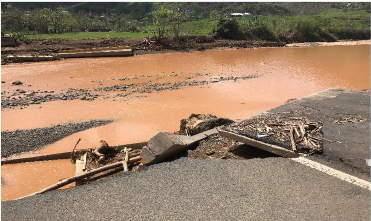
Figure 2-225: Inspection of collapsed Bridge 1462 (source: PRHTA)
