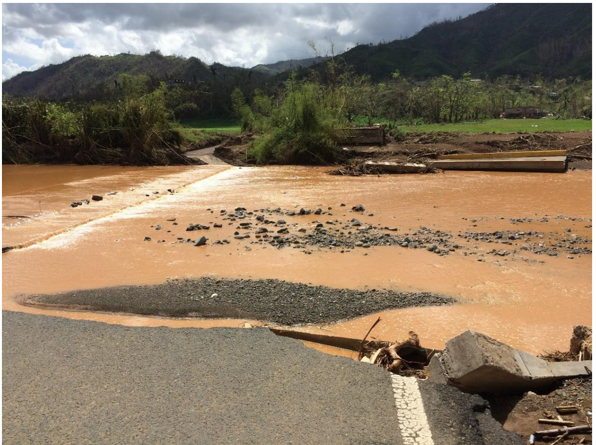
Figure 2-227: Social media image of collapsed Bridge 1462 (source: Julia Maldonado)
