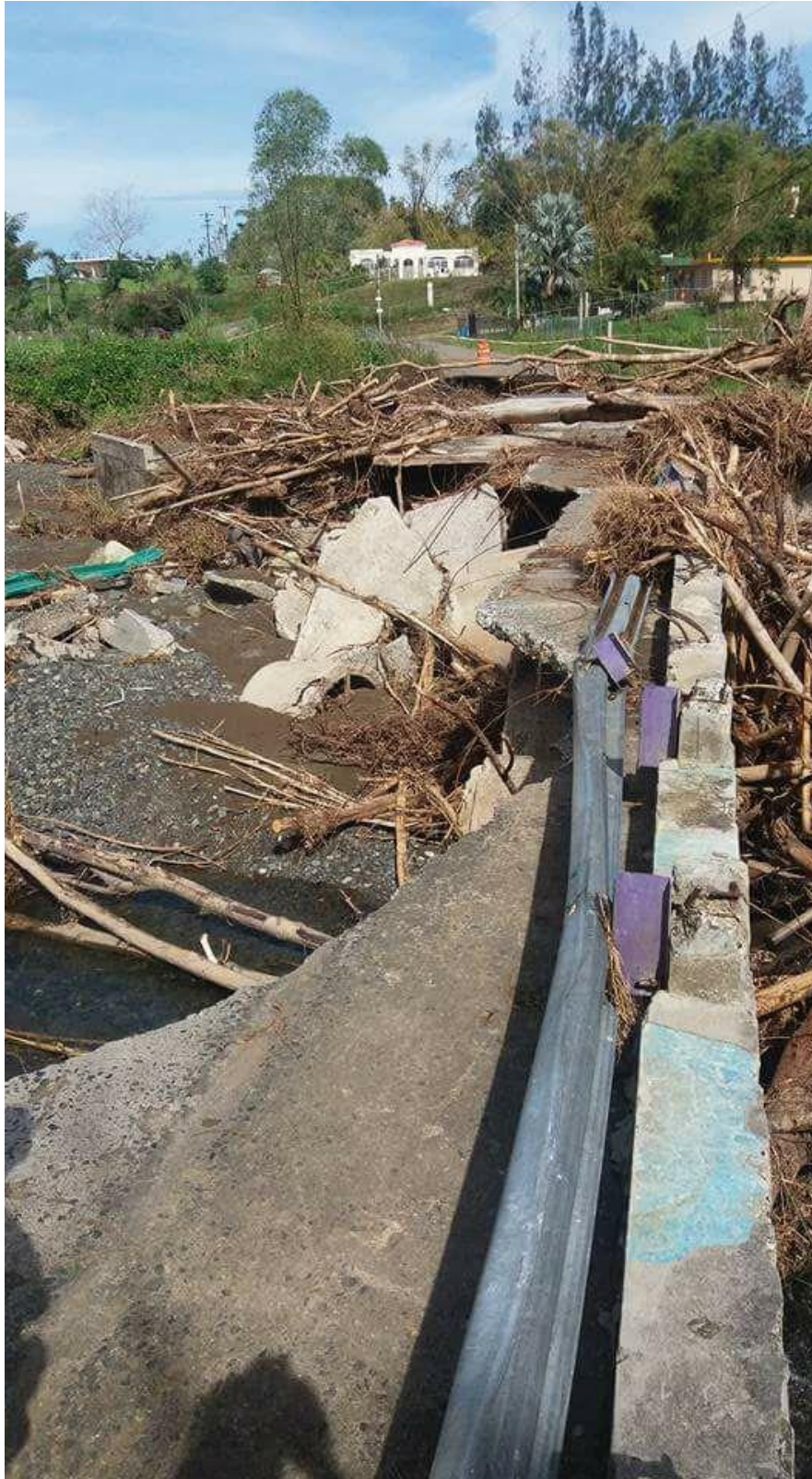
Figure 2-315: Social media image of collapsed Bridge 1728 (source: Leyda Ortiz)
