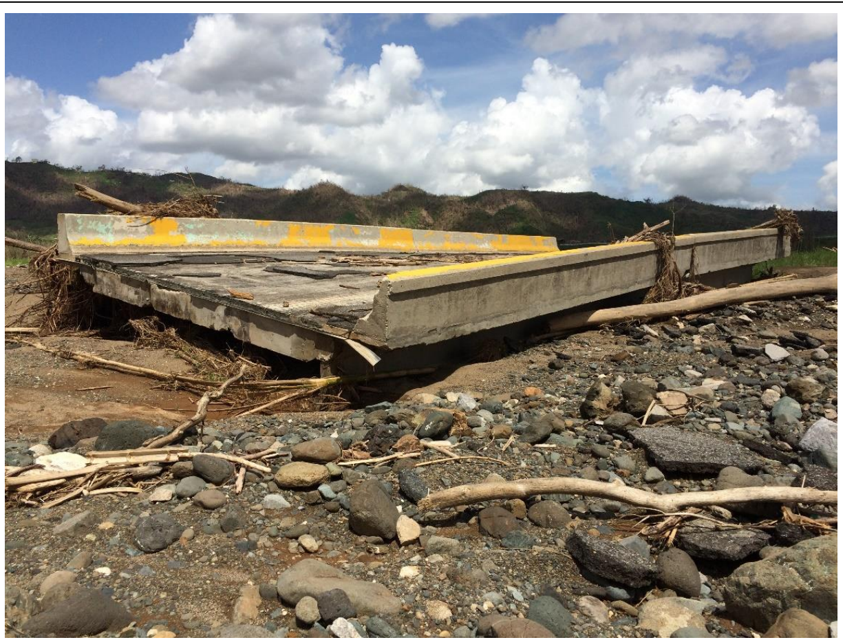
Figure 2-229: Social media image of collapsed Bridge 1462 (source: Julia Maldonado)
