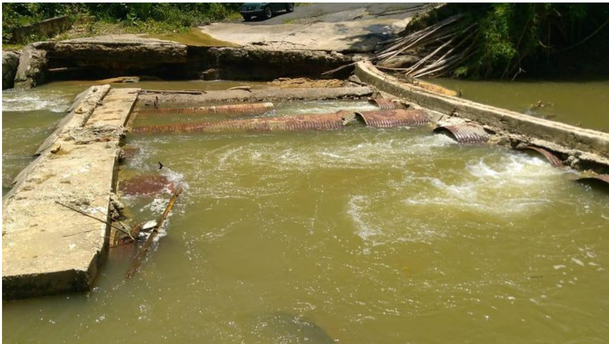
Figure 4-30: News report image of collapsed Bridge Seis Bocas (source: El Nuevo Día)
