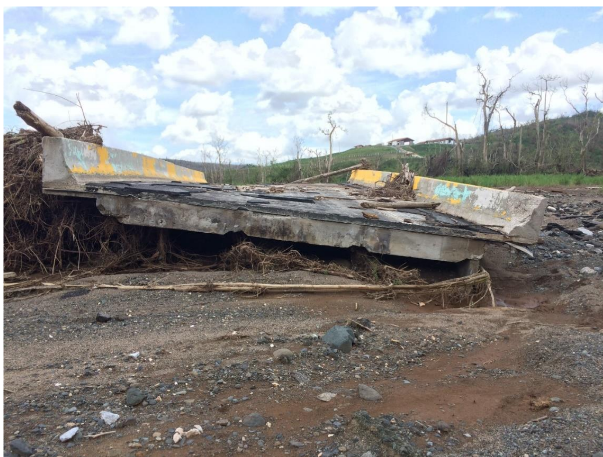
Figure 2-228: Social media image of collapsed Bridge 1462 (source: Julia Maldonado)
