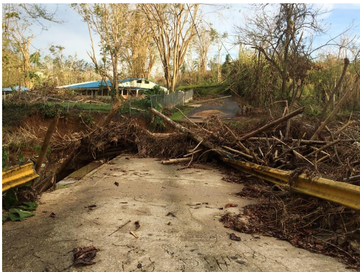
Figure 3-60: Social media image of collapsed approach of Bridge 1684 (source: Julia Maldonado)
