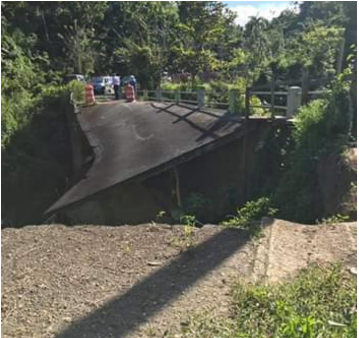
Figure 4-22: Social media image of collapsed La Riviera Sector Bridge (source: Rafael June Rivera)
