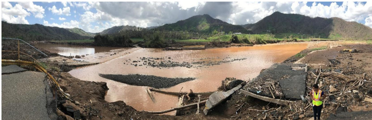
Figure 2-221: Inspection of collapsed Bridge 1462 (source: PRHTA)
