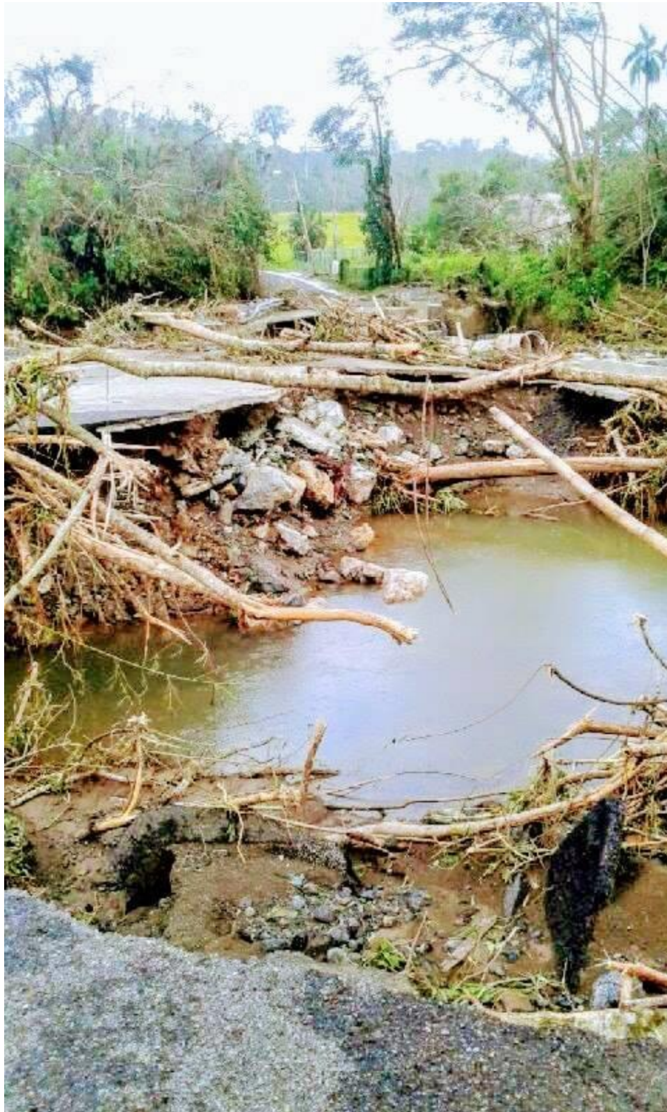
Figure 2-314: Social media image of collapsed Bridge 1728 (source: Coleccionistas Coampi)
