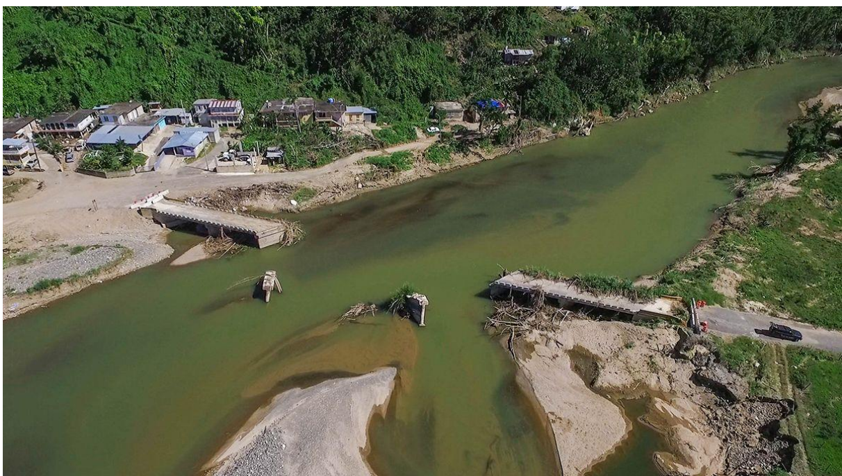
Figure 2-364: Social media image of collapsed Bridge 1917 (source: Mabey Bridge)
