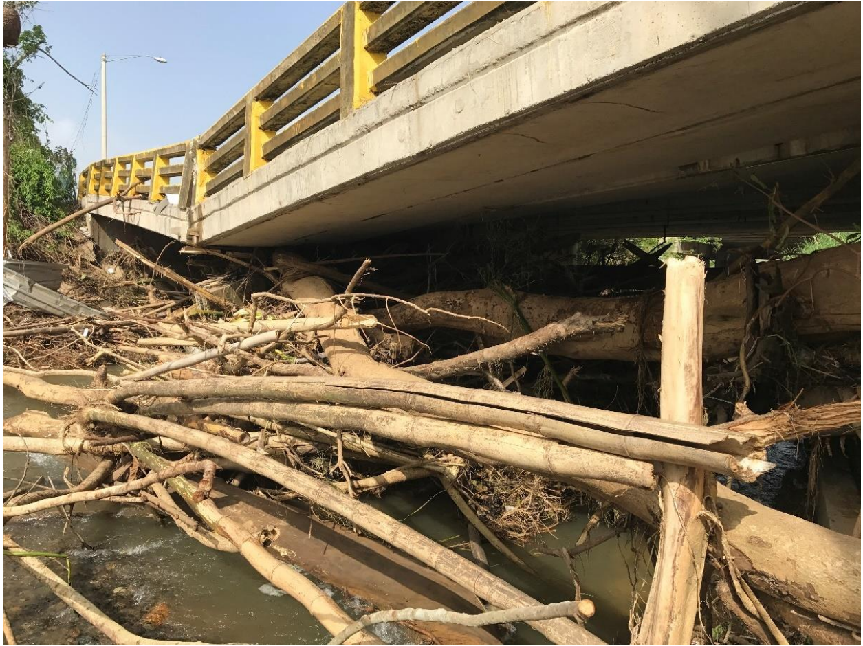
Figure 2-195: Image of damaged Bridge 1453 (source: PRHTA)
