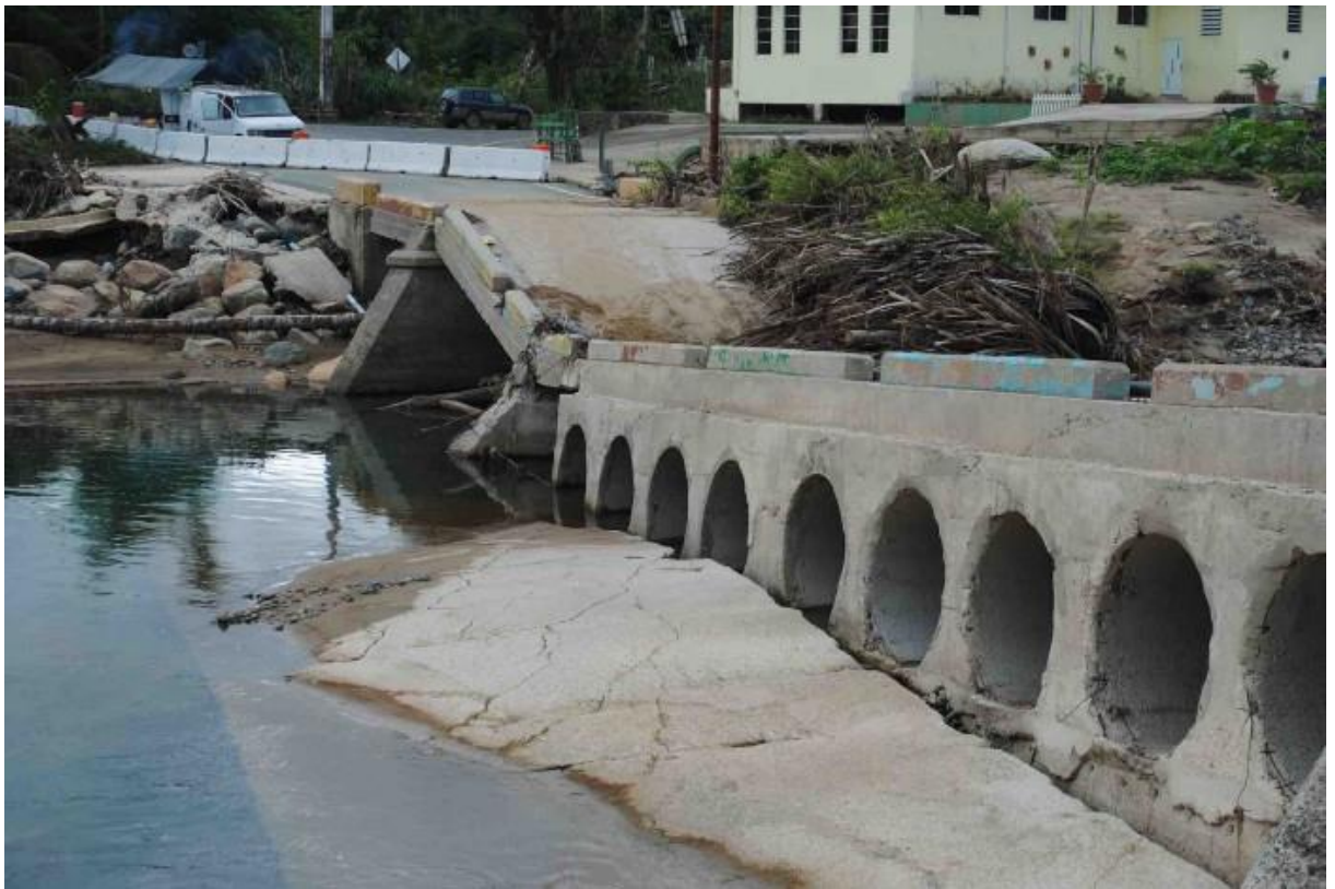
Figure 2-22: Social media image of collapsed Bridge 505 (source: Robert L. Read)
