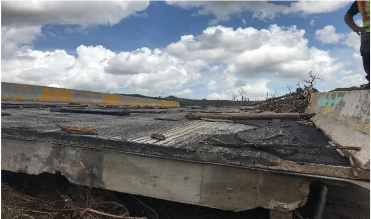
Figure 2-224: Inspection of collapsed Bridge 1462 (source: PRHTA)
