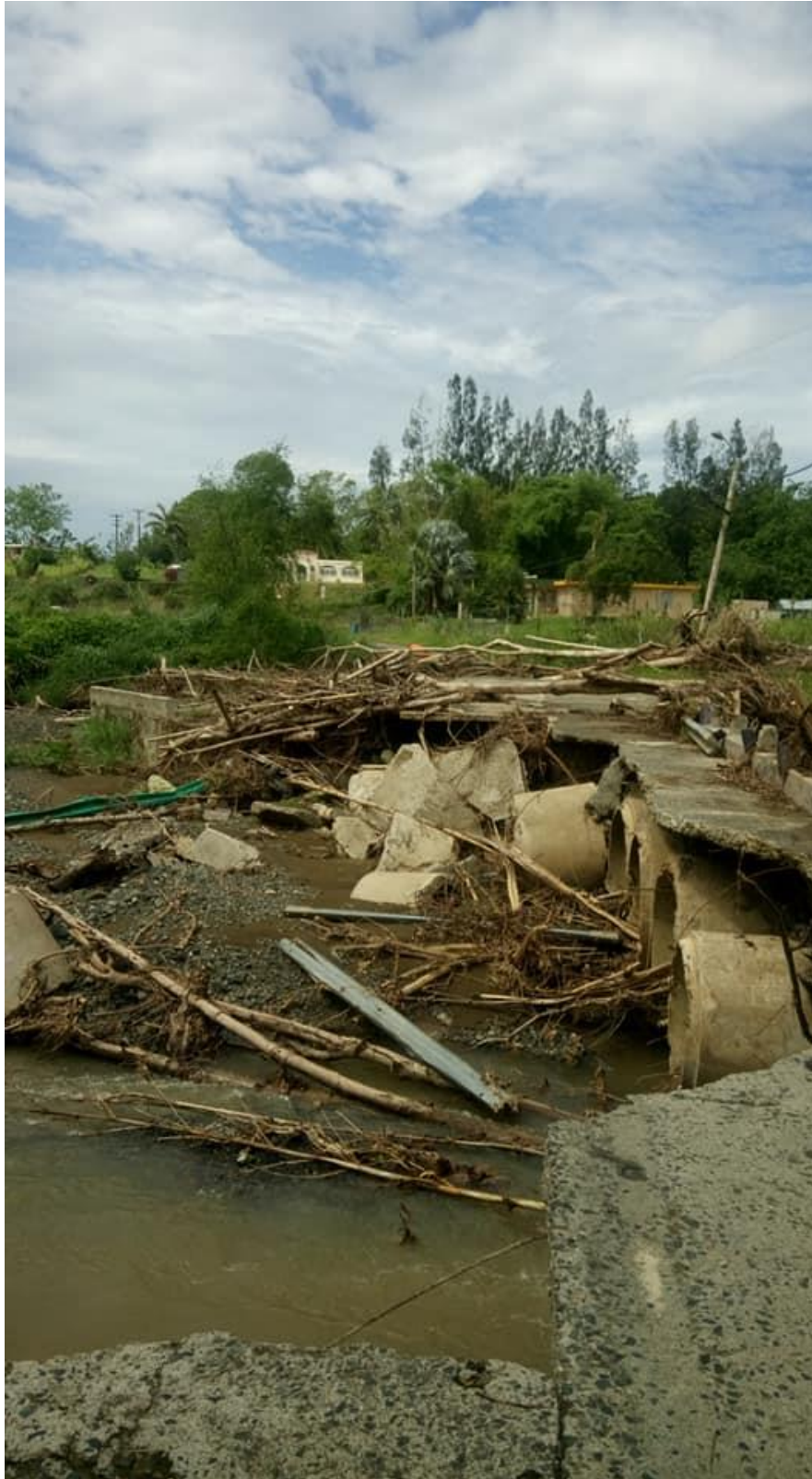
Figure 2-316: Social media image of collapsed Bridge 1728 (source: Miriam Cruz Miranda)
