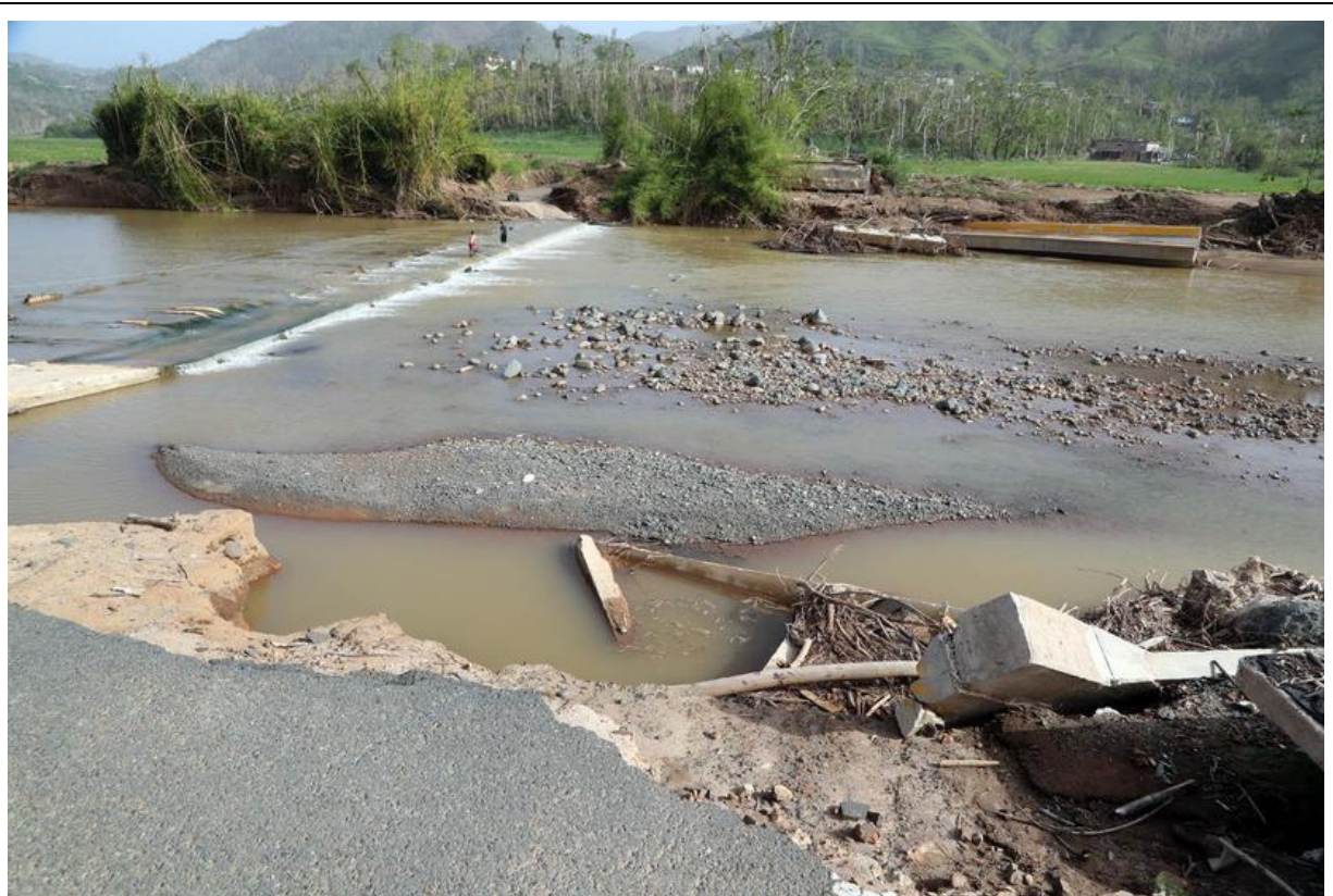
Figure 2-236: Collapsed Bridge 1462 image from news report (source: El Nuevo Día)
