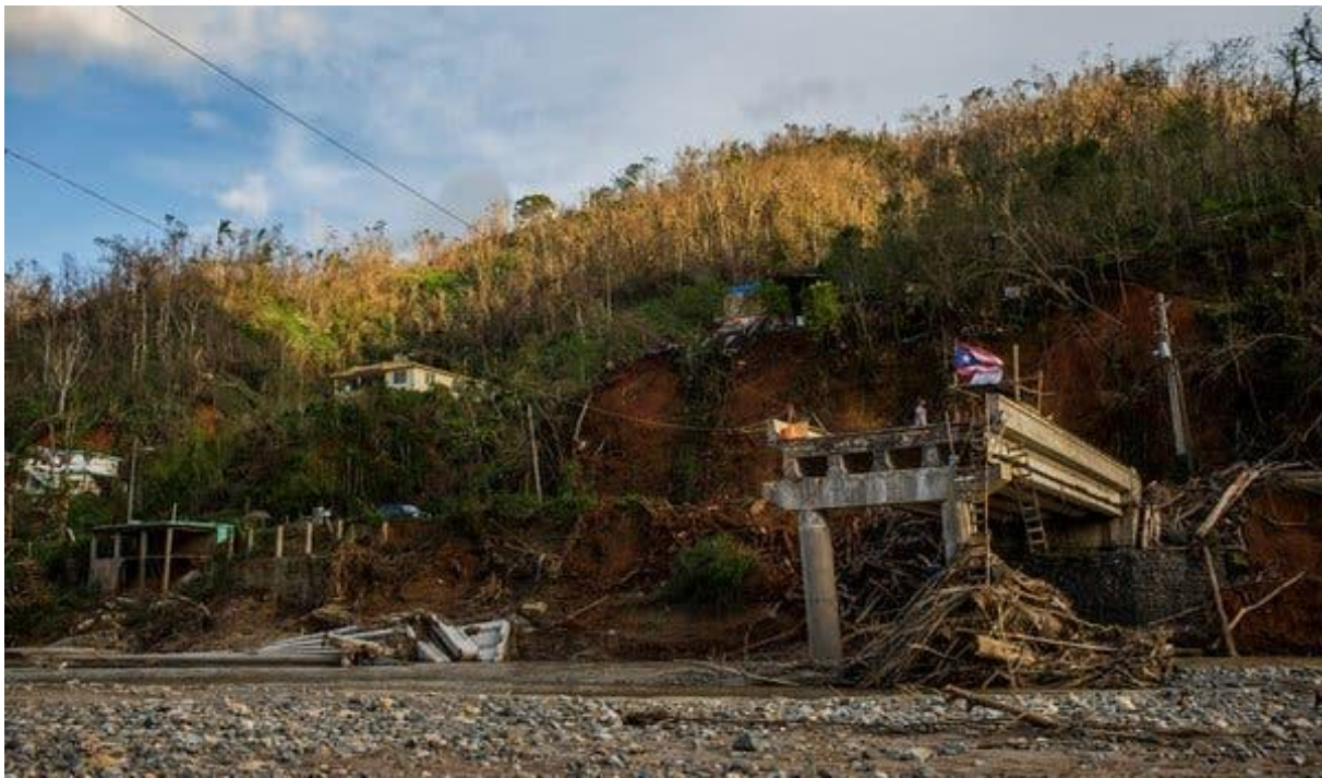
Figure 2-266: News report image of collapsed Bridge 1499 (source: NY Times)
