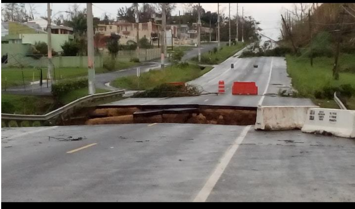
Figure 2-334: Social media image of collapsed Bridge 1733 (source: Joaquín Lebrón Rosado)
