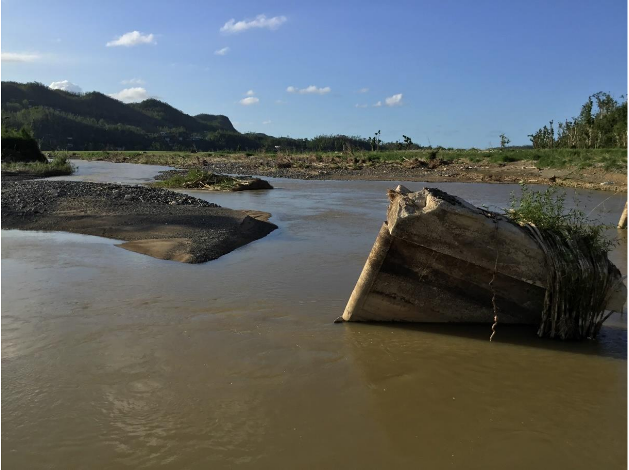
Figure 2-357: Collapsed Bridge 1917 (source: PRHTA)
