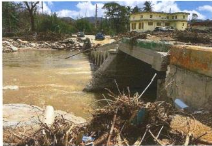
Collapsed Low Bridge from North Abutment Downstream
