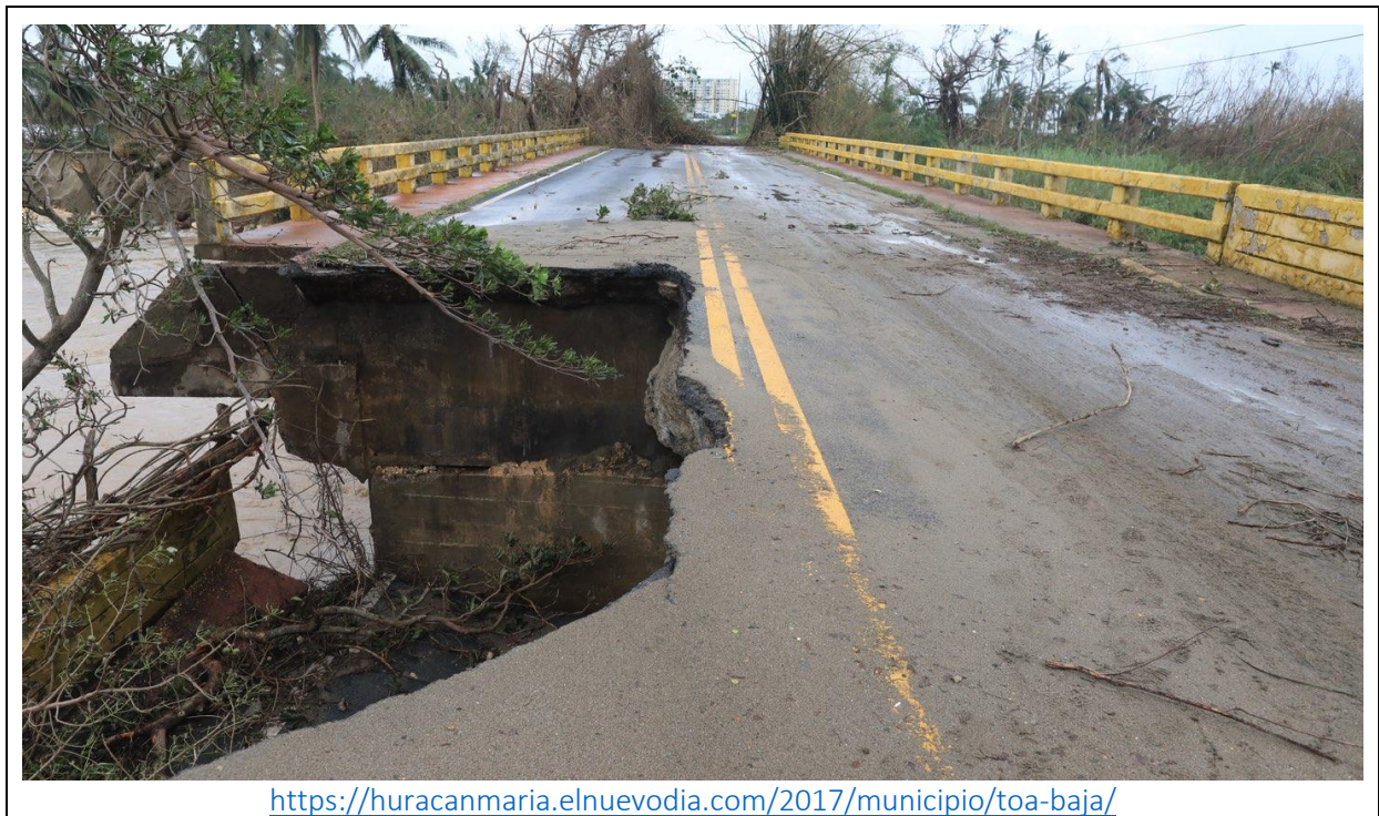
Figure 3-24: News report image of partial collapse of approach of Bridge 635 (source: El Nuevo Día)
