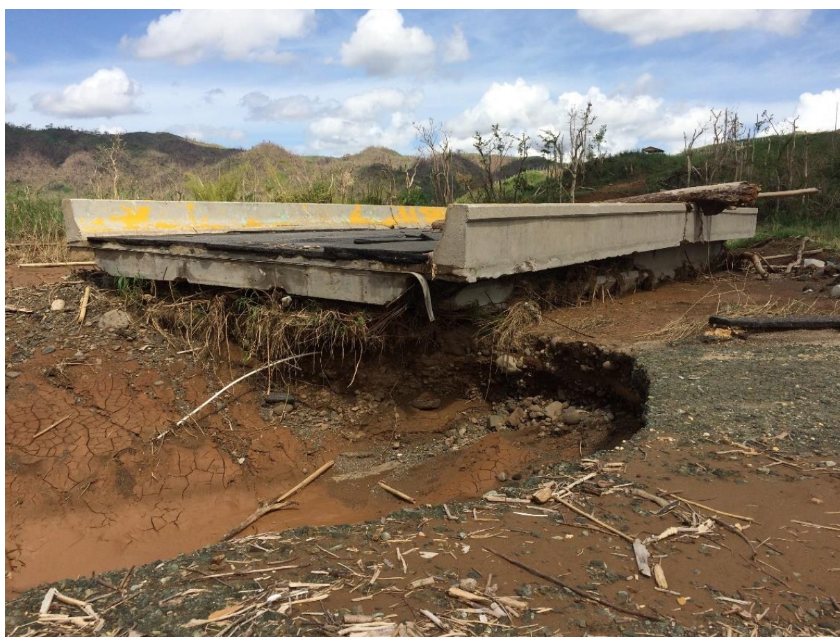
Figure 2-230: Social media image of collapsed Bridge 1462 (source: Julia Maldonado)
