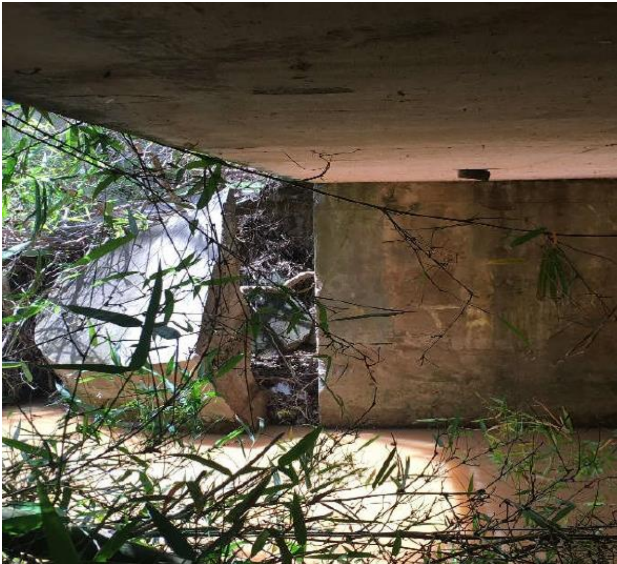
Figure 5-12: Photo of collapsed wingwall of Bridge 1629 taken during October 20,2017 inspection (source: PRHTA)
