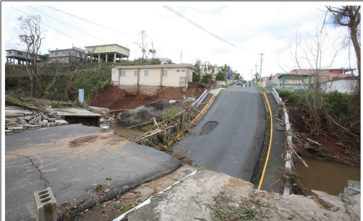
Figure 2-284: Collapsed Bridge 1698 image from news report (source: El Nuevo Día)
