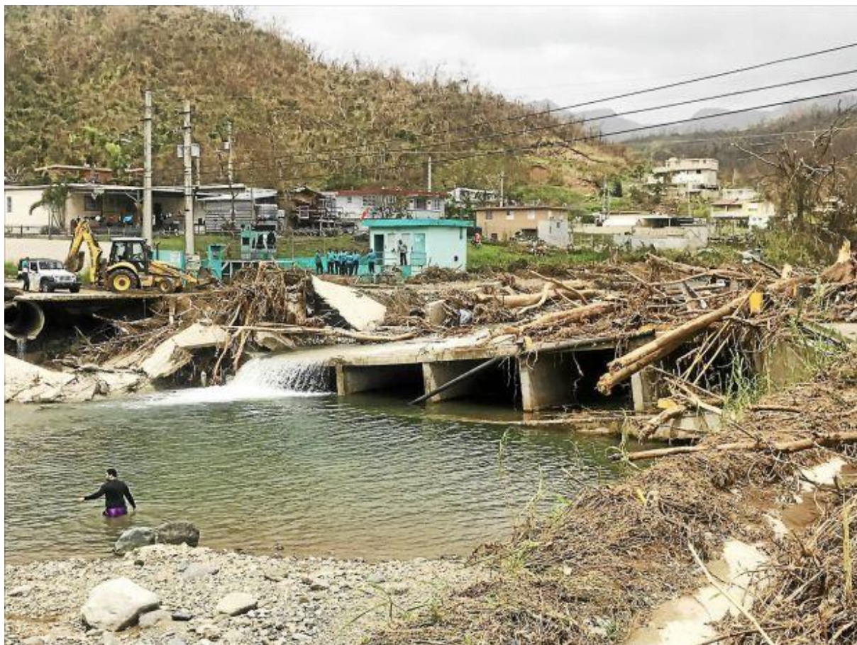
Figure 2-429: News report image of collapsed Bridge 2842 (source: Héctor Martínez)
