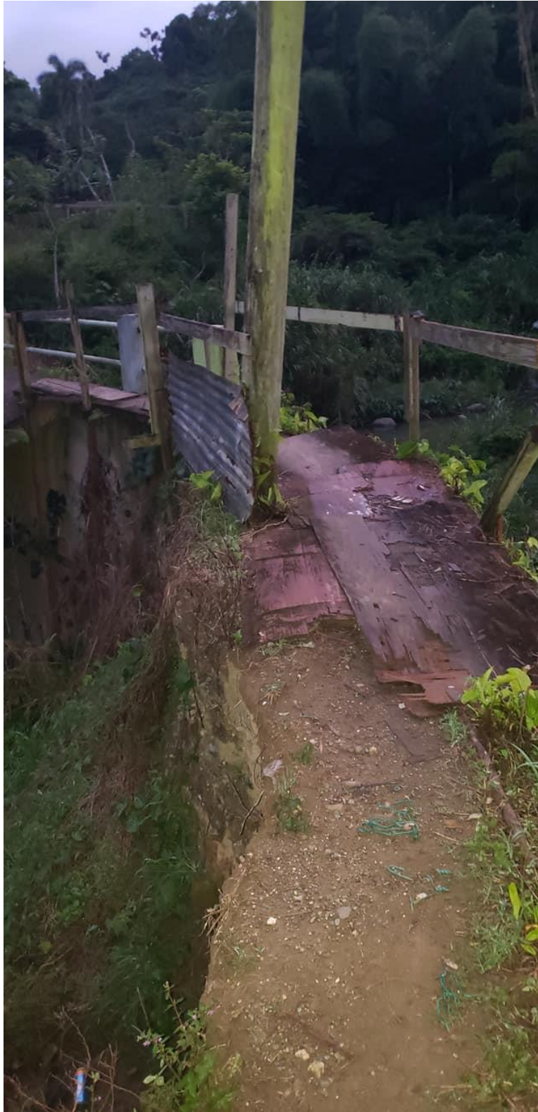
Figure 4-24: Social media image of collapsed La Riviera Sector Bridge (source: Geovanny Torres Rivera)
