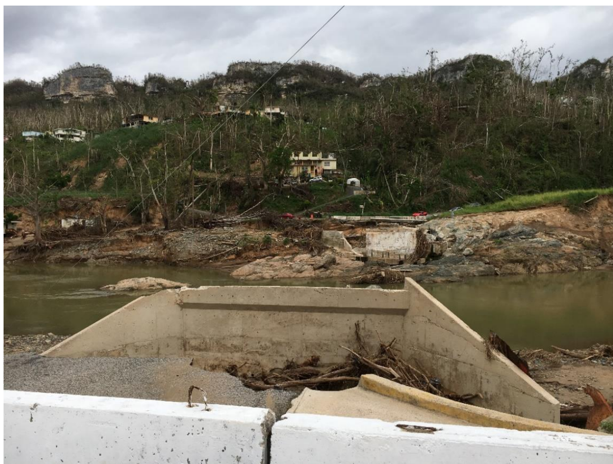
Figure 2-119: Social media image of collapsed Bridge 1130 (source: Julia Maldonado)
