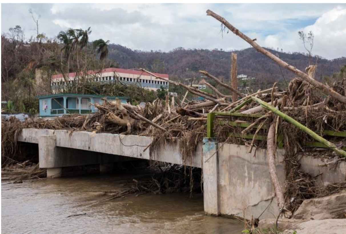
Figure 5-13: Debris accumulation in a bridge in Utuado (source: NBC News)
