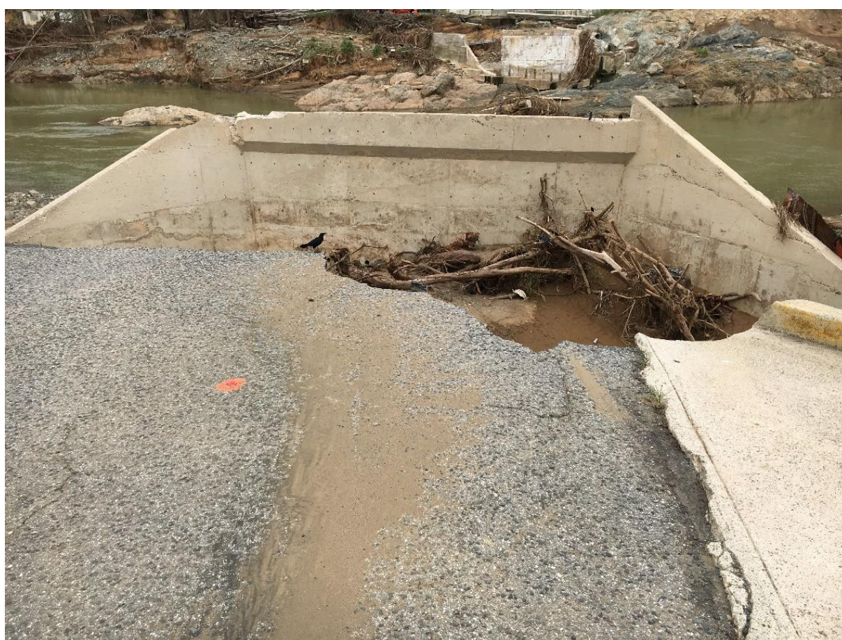
Figure 2-117: Social media image of collapsed Bridge 1130 (source: Julia Maldonado)
