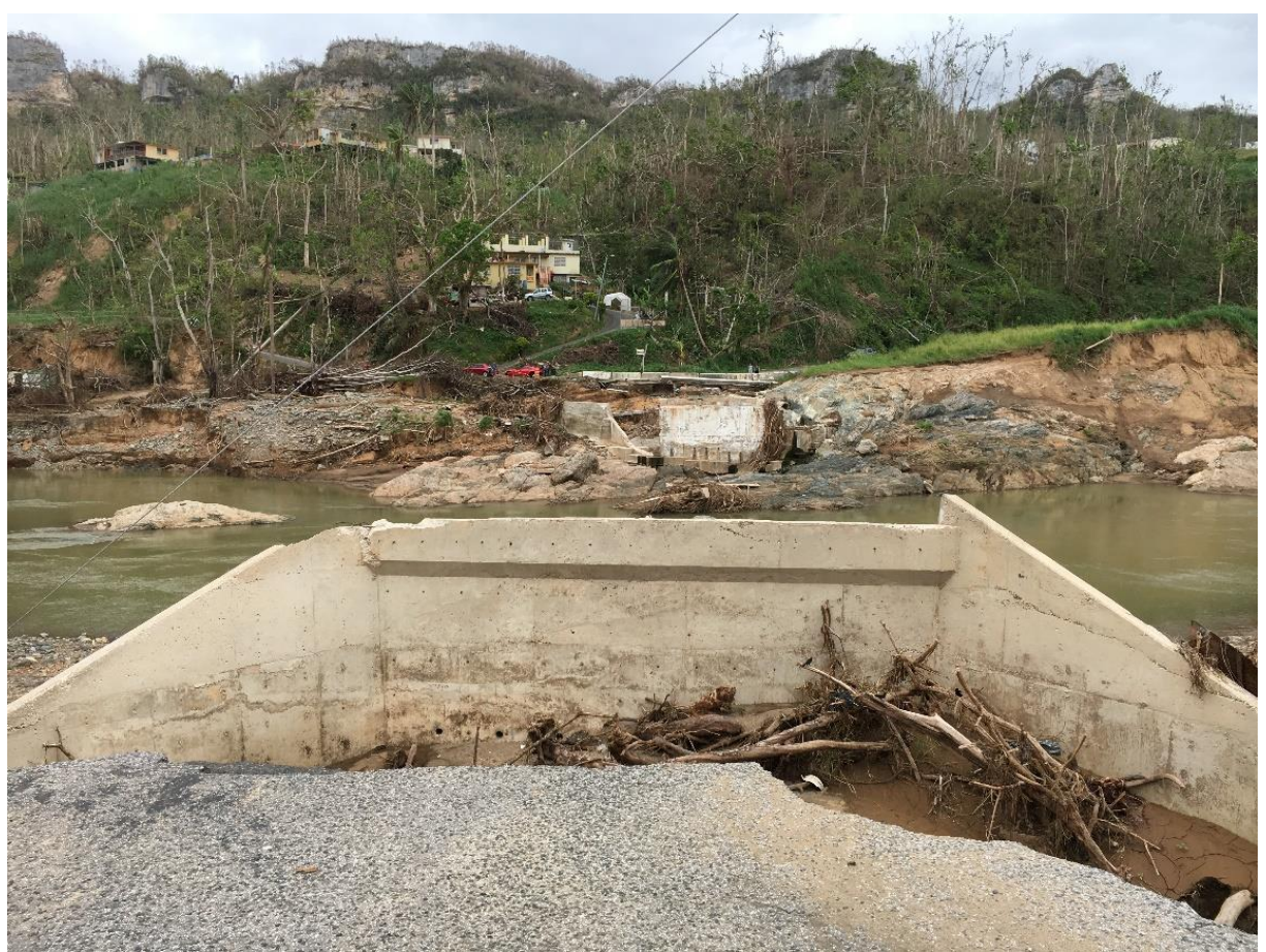
Figure 2-118: Social media image of collapsed Bridge 1130 (source: Julia Maldonado)
