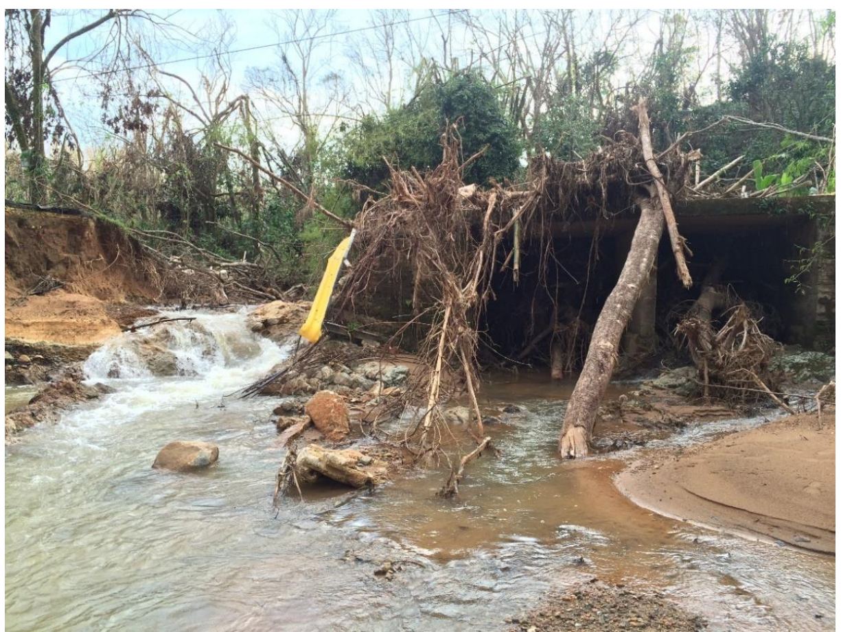
Figure 3-59: Social media image of collapsed approach of Bridge 1684 (source: Julia Maldonado)
