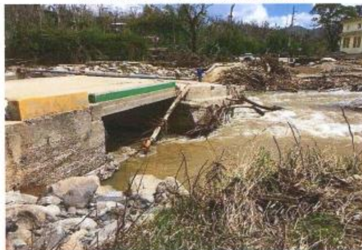
Collapsed Low Bridge from North Abutment Upstream
