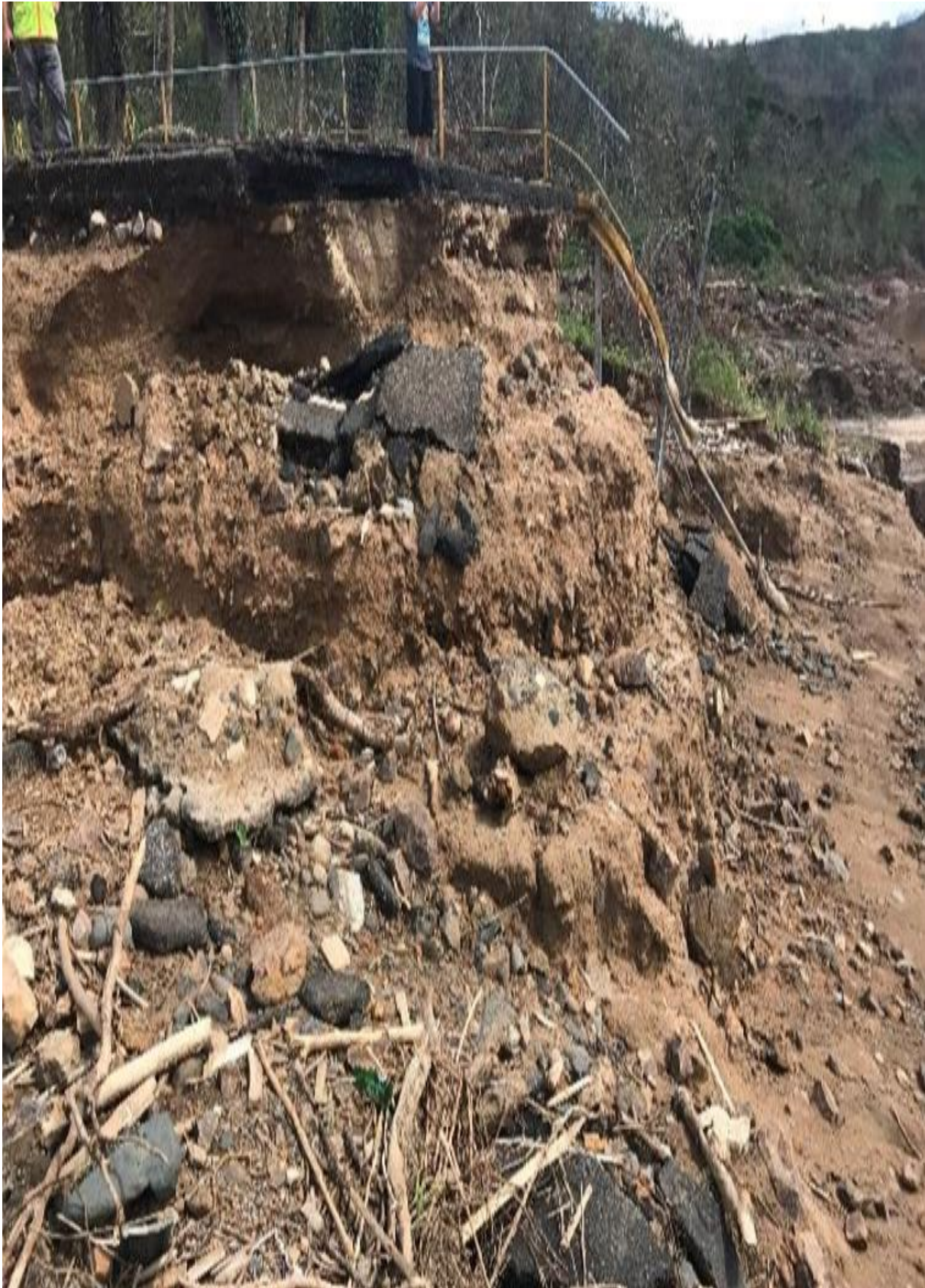
Figure 2-223 Inspection of collapsed Bridge 1462 (source: PRHTA)
