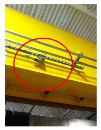
Figure 23: Structure bumper kill switch (circled)
