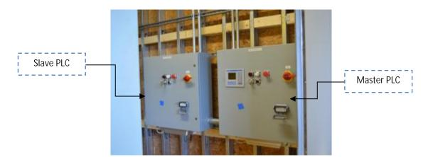
Figure 7. Rail Cart Control System
