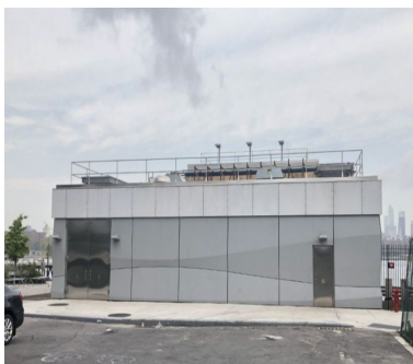
New, watertight fan plant exterior above Canarsie Tube
