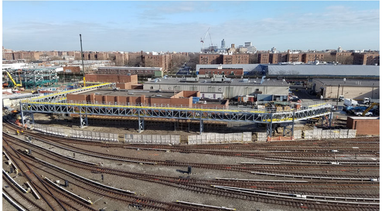
Elevated cable bridge at Coney Island Yard
