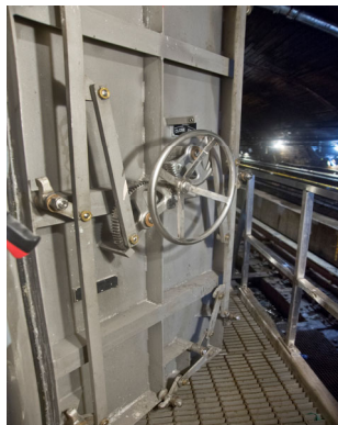
Marine door at Montague Tube circuit breaker house
