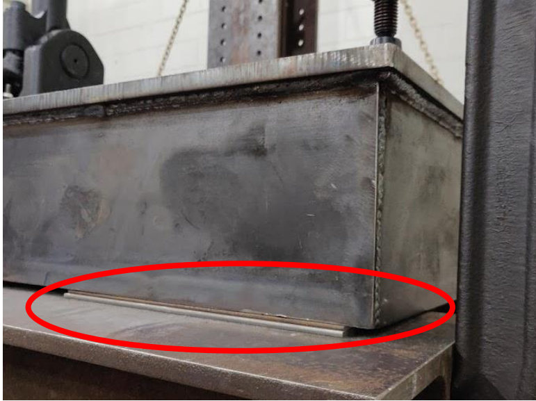
Figure 4 Shims to support deck edge
