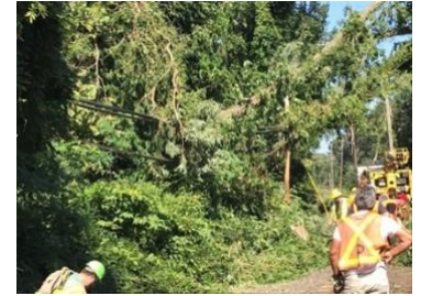
Photo @ Metropolitan Transportation Authority
