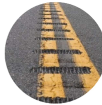
Local Safety Program/High Risk Rural Road $22 Million
